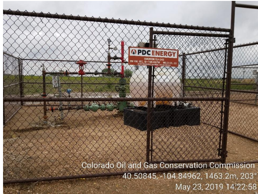
Photo 1: Wellhead w/methanol pump
