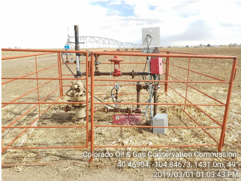
Photo #3 HCW 24-23 (05-123-31497) Wellsite Shut-In | SI Emergency number NOT posted Sign not attached from prior insp.
