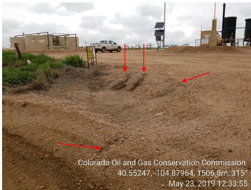
Photo 5: Erosion at entrance of loction.
