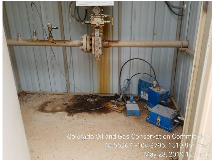
Photo 6: Trash/unused equipment inside east gas meter house/oily waste.
