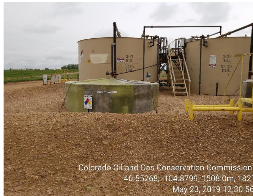
Photo 2: No BBLS on South produced water tank.
