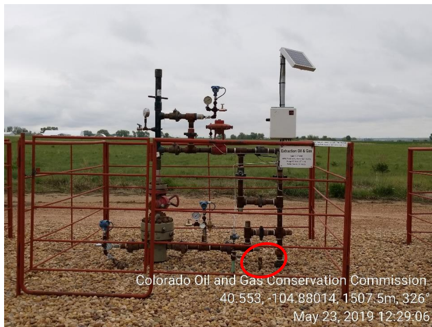
Photo 1: Wellhead; UNUSED RISER
