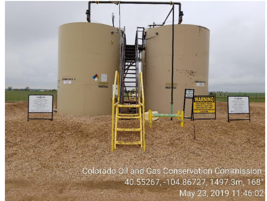
Photo 2: Centralized Tank Battery
