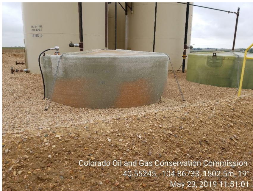
Photo 3: No BBLs on produced water tank.
