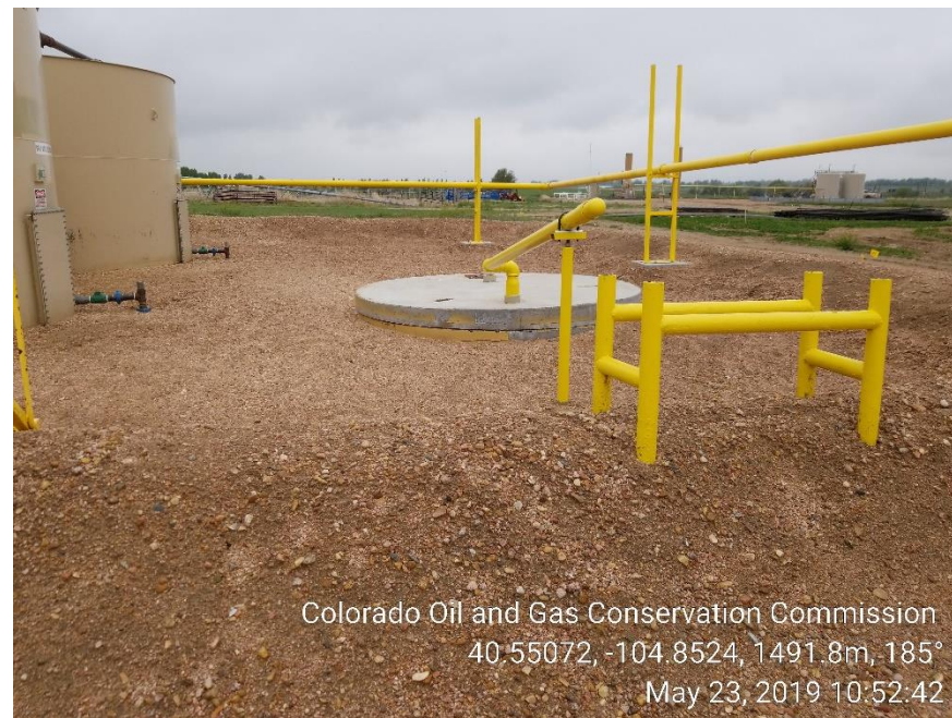
Photo 2: NO SIGNAGE for produced water tank or placard
