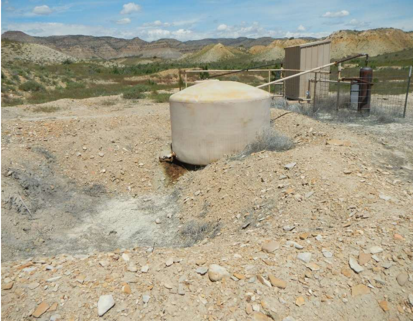
Photo #3 – Oil stained soil beneath the valve on the produced water tank. Pit 119480 located southwest of the produced water tank. Photo taken looking north
