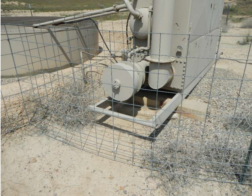
Photo #5 – Vegetation around horizontal heated separator.
