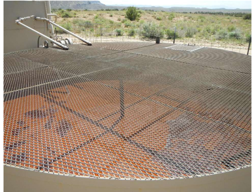
Photo #8 – View of 95 bbl partly buried produced water tank fluids.
