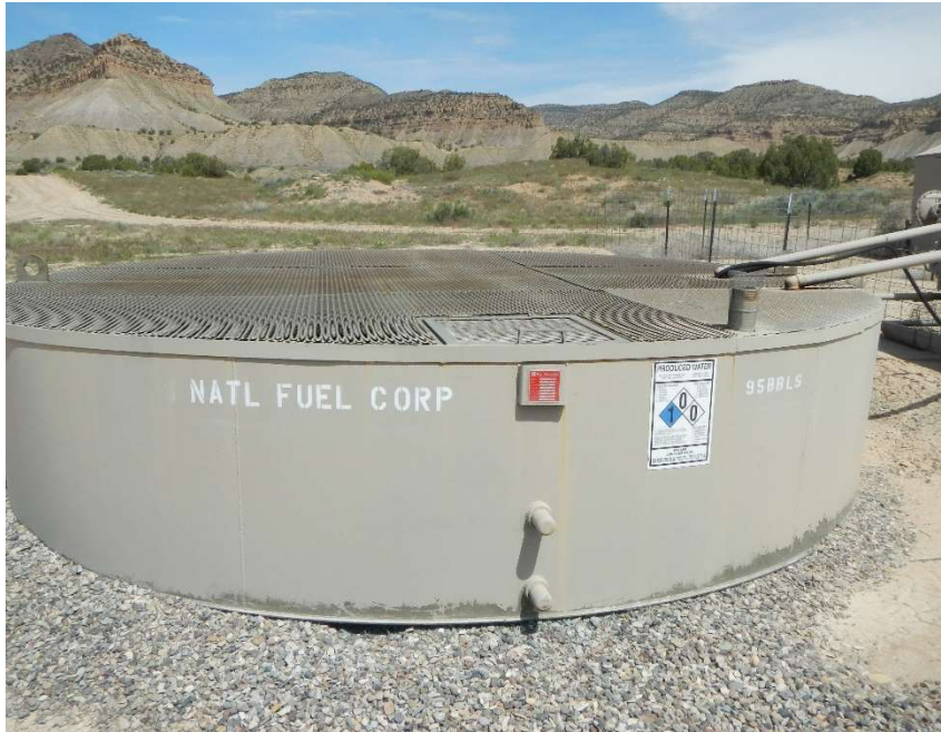
Photo #7 – View of 95 bbl partly buried produced water tank looking north.
