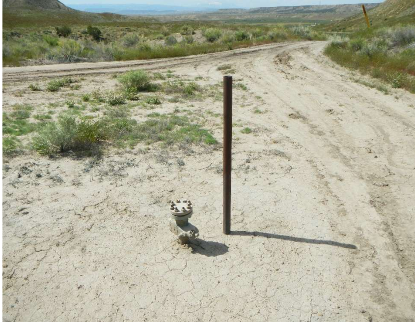
Photo #3 – View of a unmarked flowline riser looking southwest.
