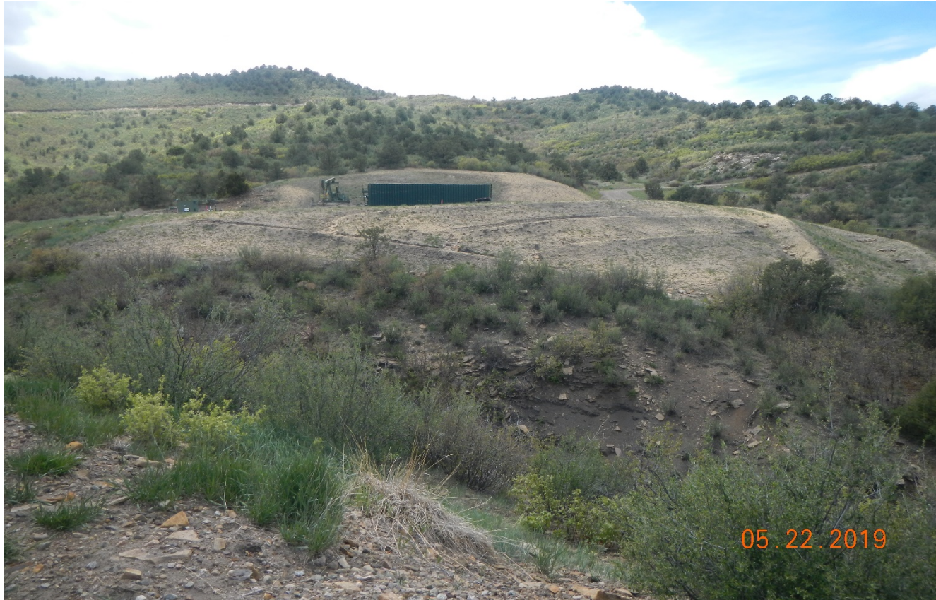
Photo 1. Facing south toward the location. The fill and cut slopes have been seeded and hydromulched.
