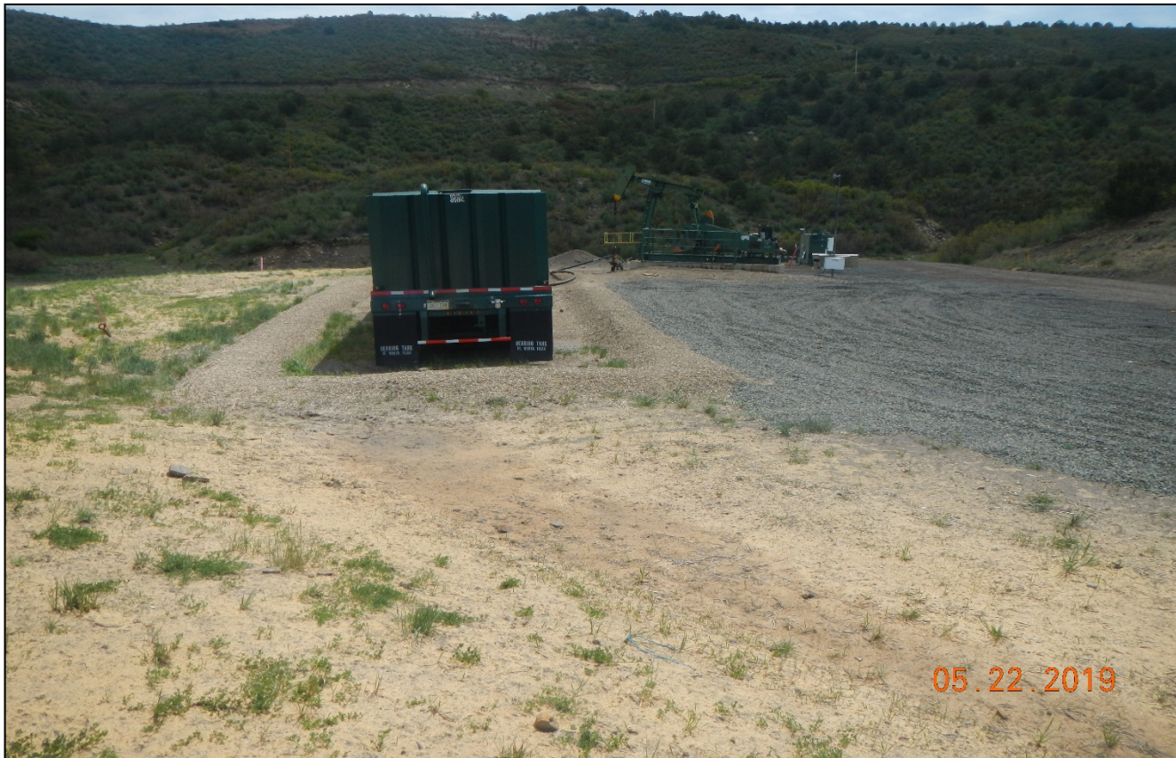
Photo 5. Gravel has been placed on pad surface. Berm is adequate around tank.
