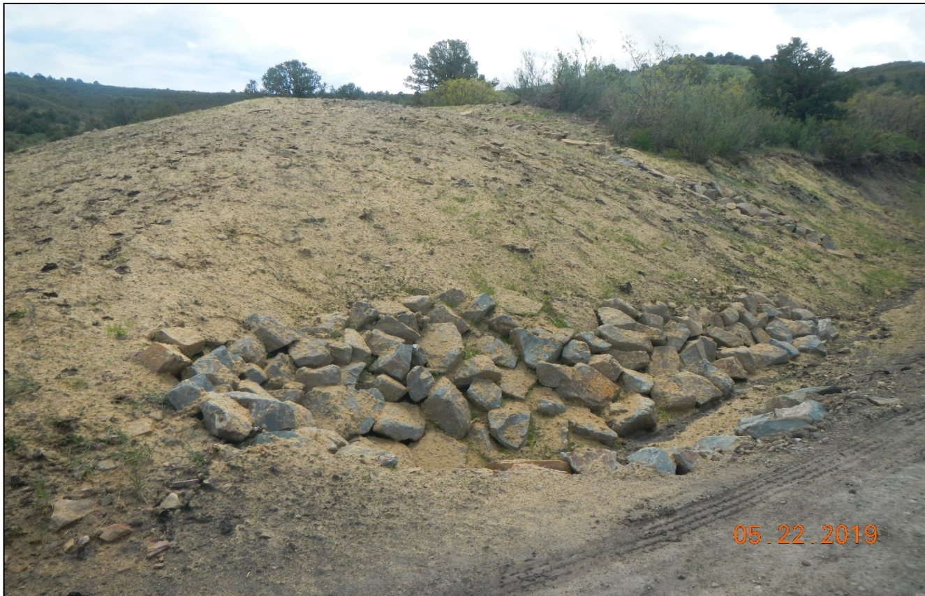
Photo 3. The cut slope has been stabilized with hydro mulch and rock rip/rap.
