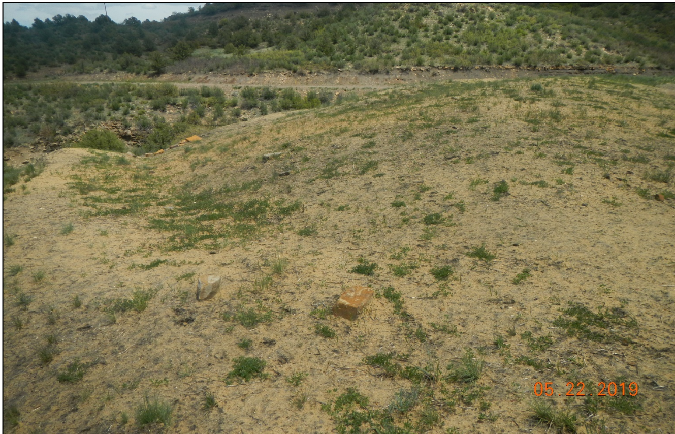
Photo 4. The fill slope has been hydromulched and seeded.
