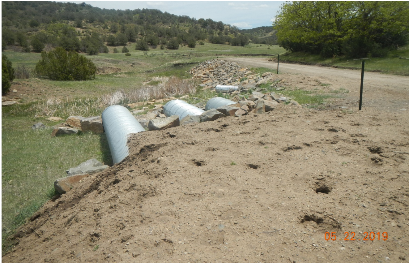
Photo 1. New culverts and rock rip/rap were installed along the main road.
