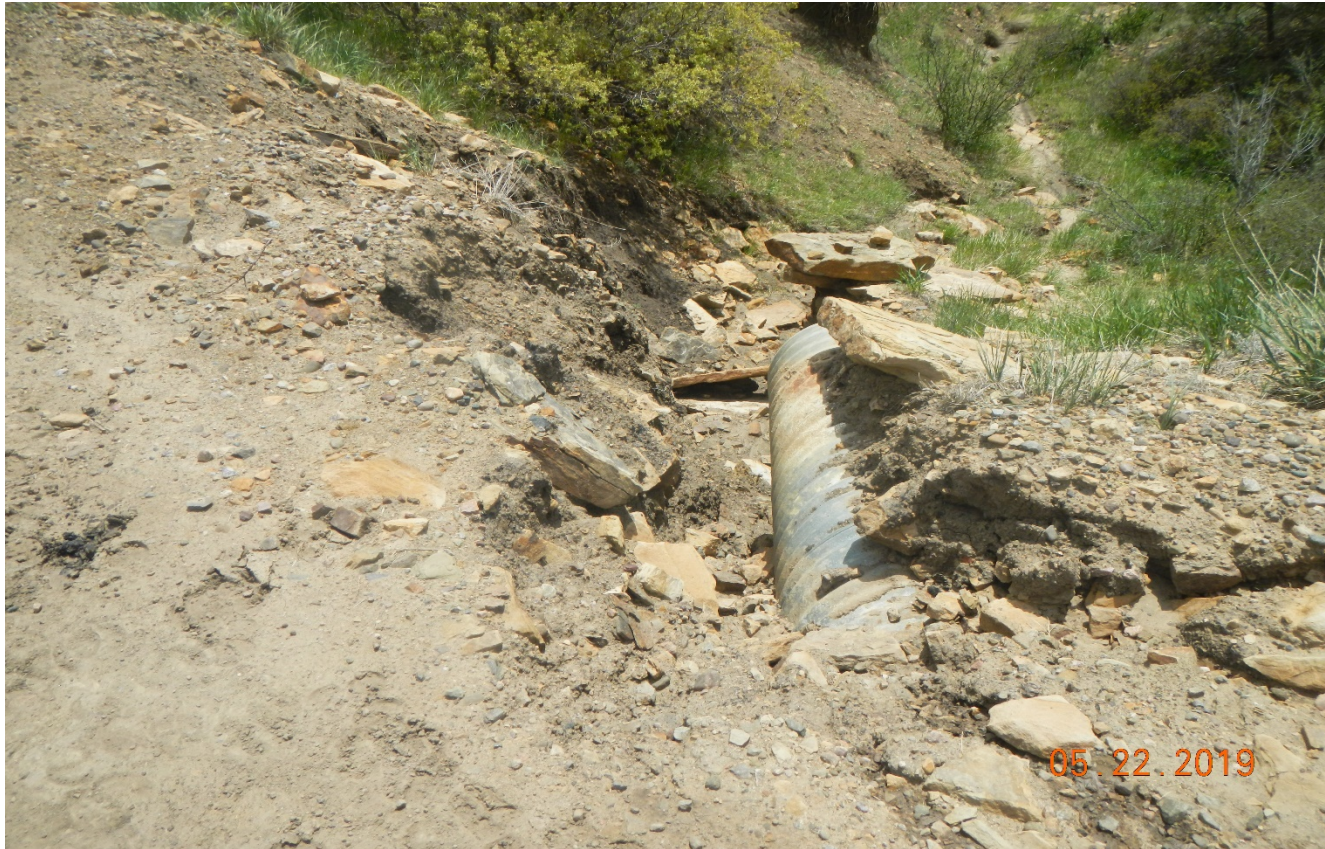
Photo 1. There is erosion issues at this outlet culvert at Lat/Long:37.09868,-104.74486. No outlet protection.
