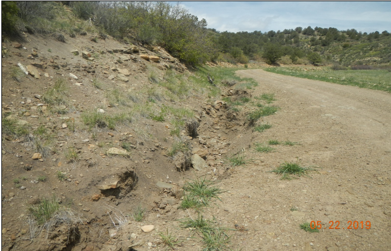
Photo 3. There is erosion channel along the access road at Lat/Long: 37.09935, - 104.74298.
