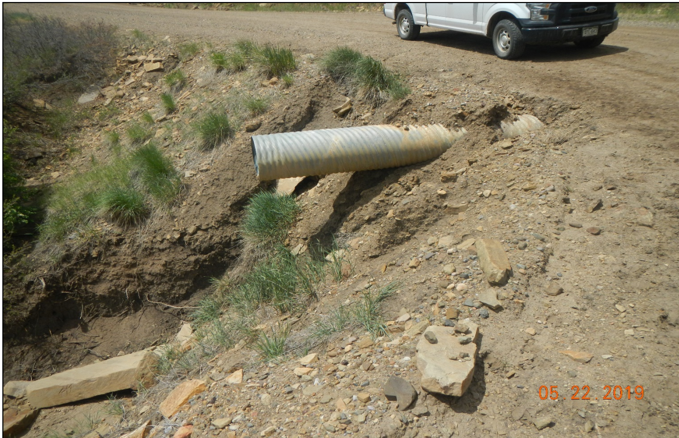
Photo 2. View of erosion around the culvert.
