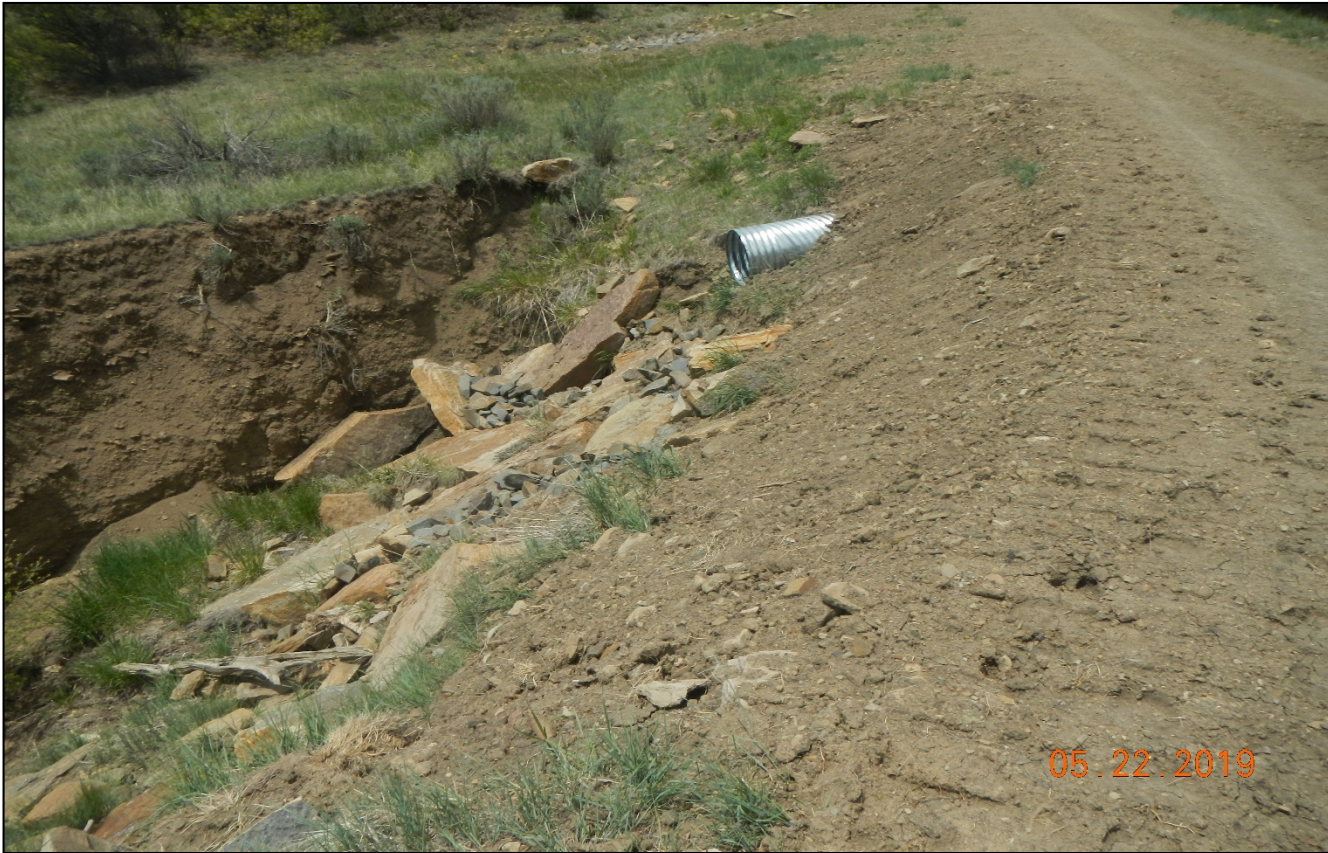
Photo 2. Rock rip/rap has been installed at the outlet.
