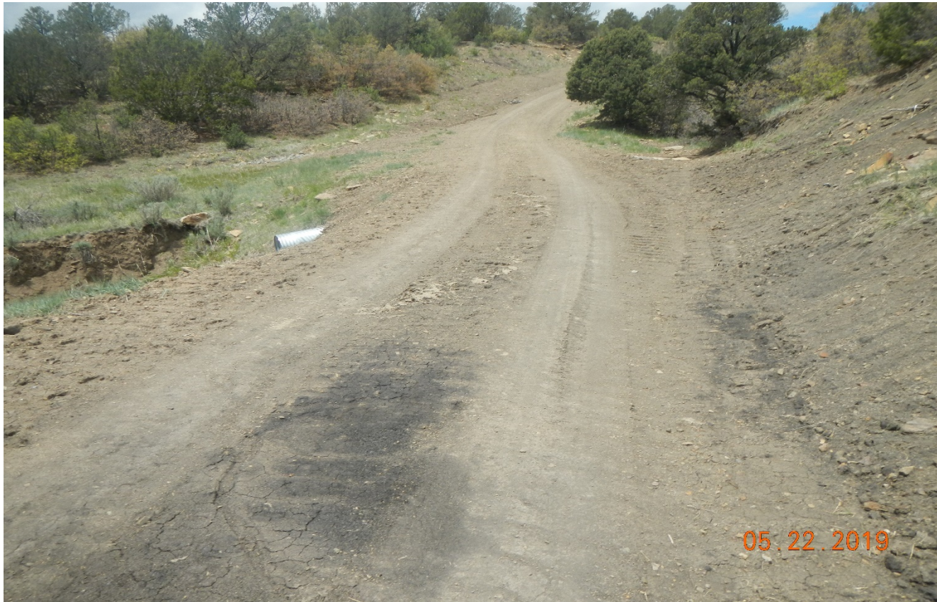
Photo 1. Facing along the access road where culvert was filled in at Lat/Long:37.09966,-104.73441. A new culvert has been installed and erosion corrected.
