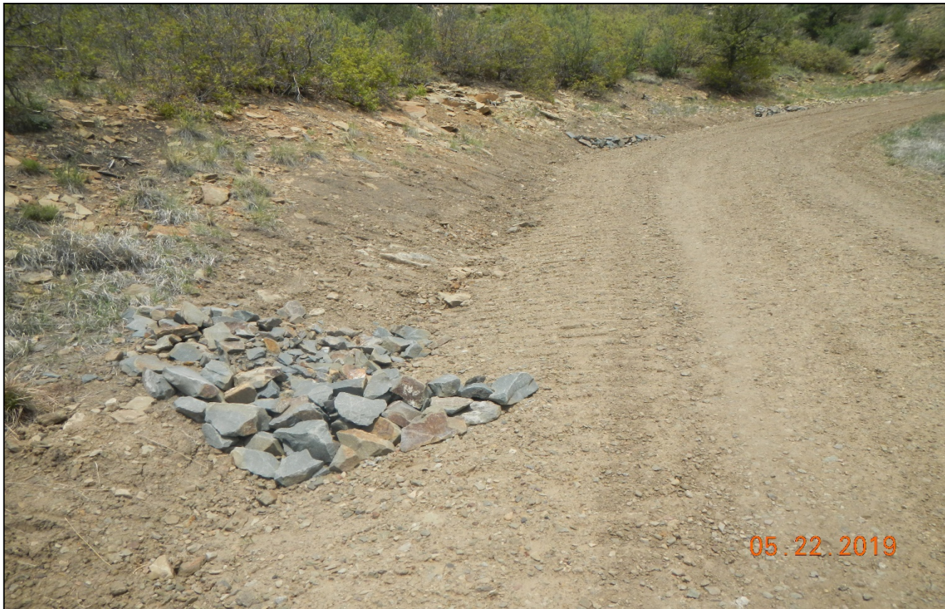
Photo 3. Rock check dams have been installed along the road.
