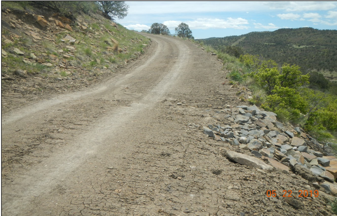
Photo 4. A water bar has been installed and the road was graded.
