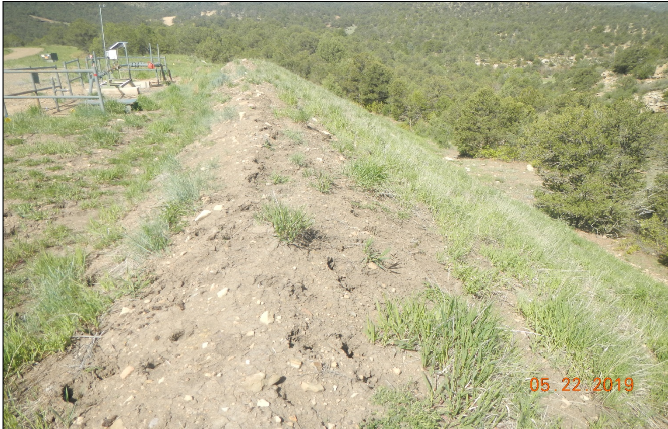
Photo 4. There is vegetation establishment along the fill slope.
