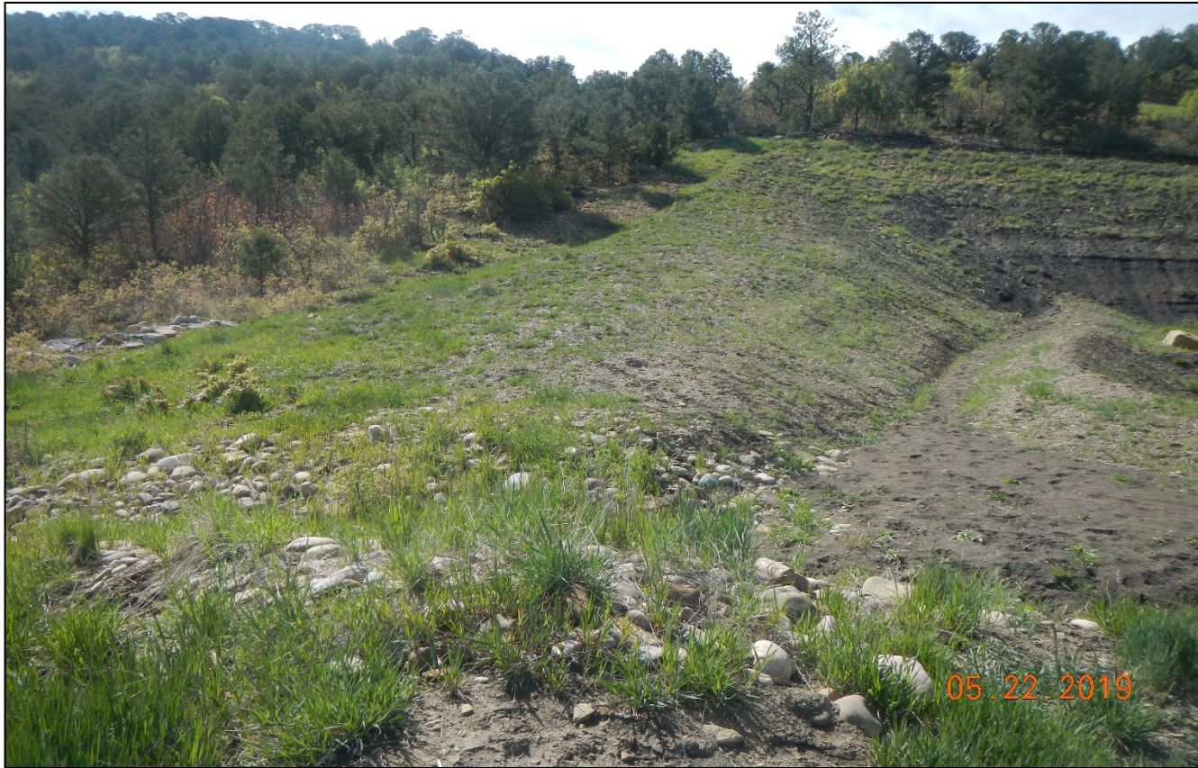
Photo 5. There is vegetation establishment along the cut slope.
