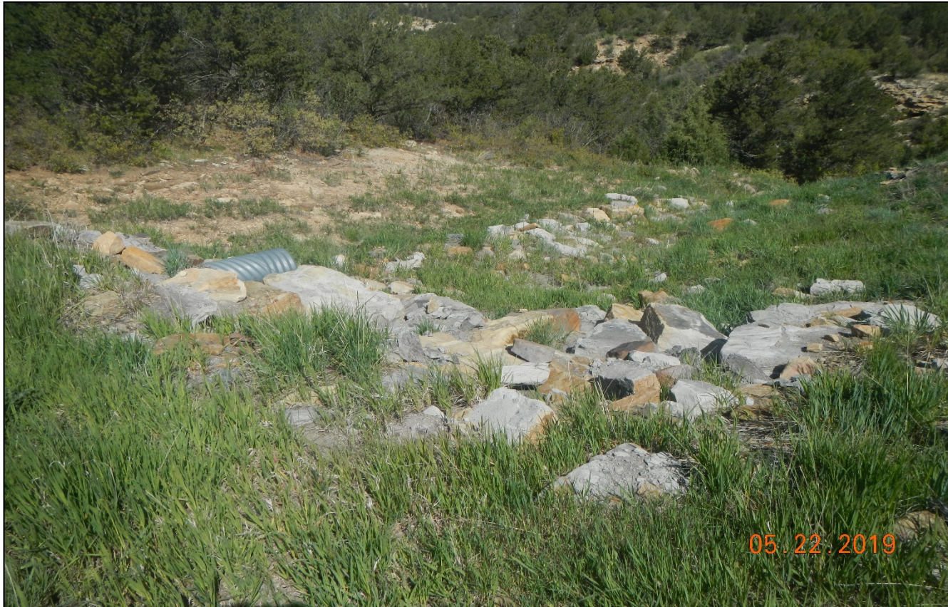
Photo 3. Outlet protection is installed at the culvert.
