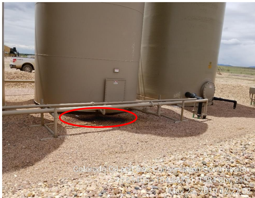
Photo 5: Stained soil behind middle crude oil tank.
