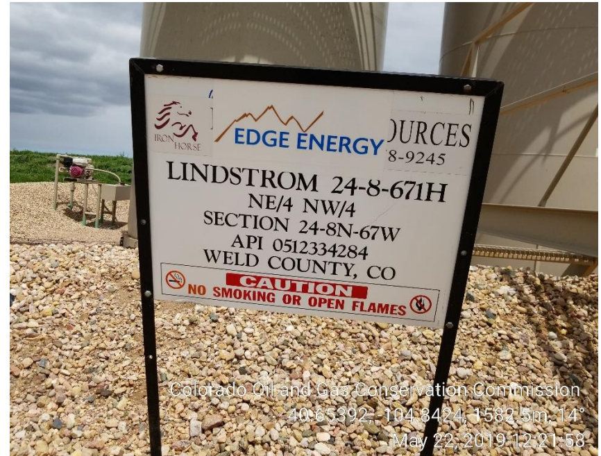
Photo 4: Tank Battery sign; MISSING EMERGENCY CONTACTS.
