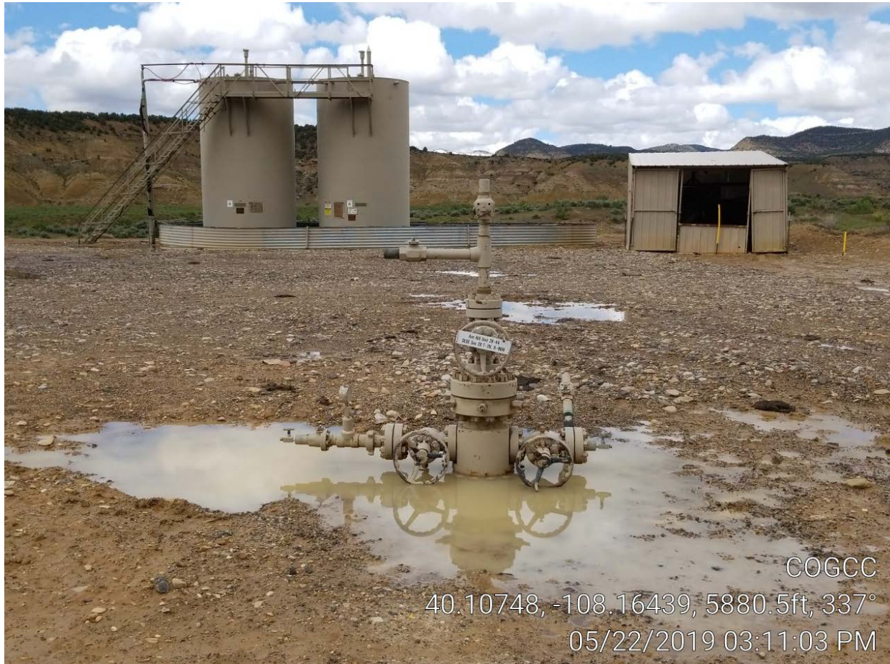
Photo 1. Location looking northwest.
