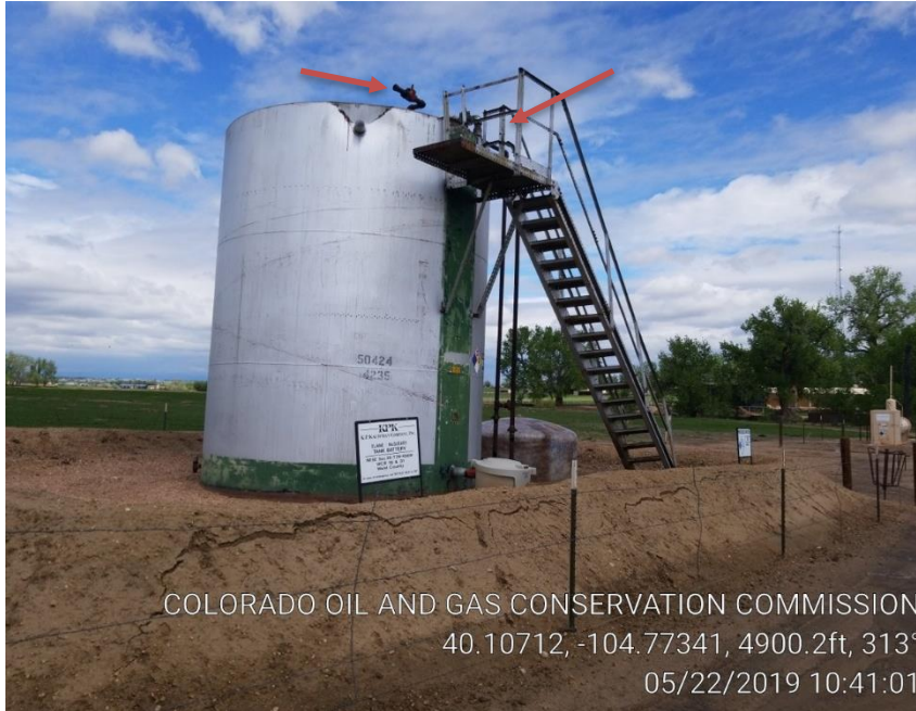
Pic 1 Tank not painted, no placard capacity, open piping not capped
