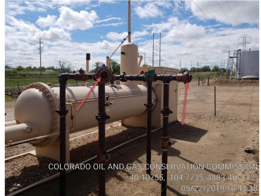
Pic 2 piping not capped on separator
