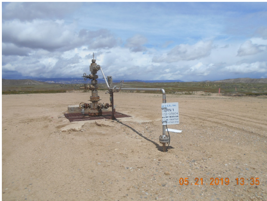
Injection wellhead
