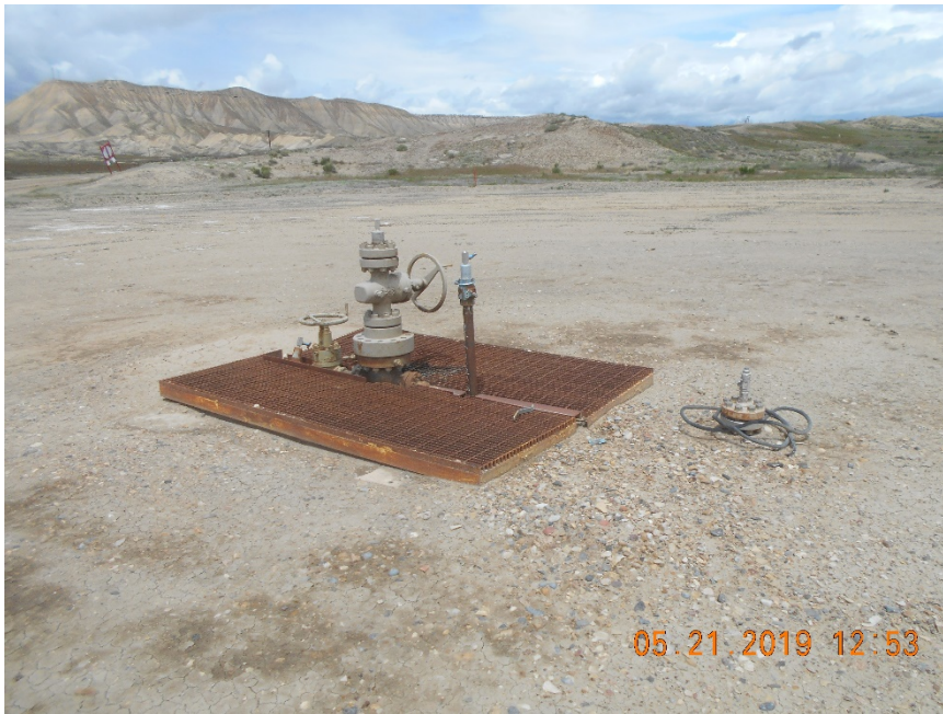
Injection wellhead
