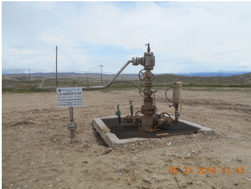
Injection wellhead
