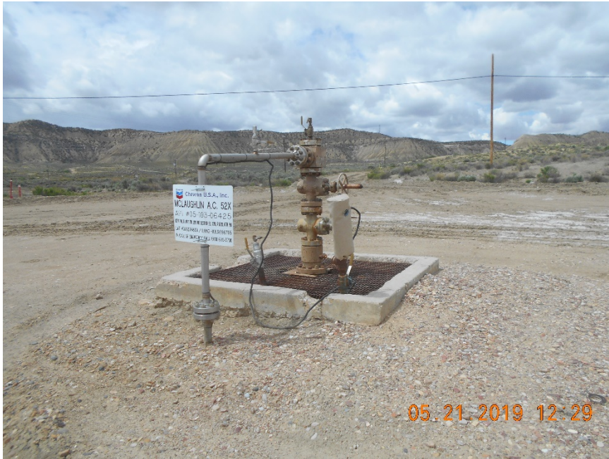
Injection wellhead
