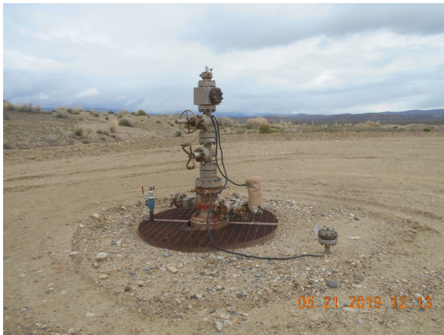
Injection wellhead
