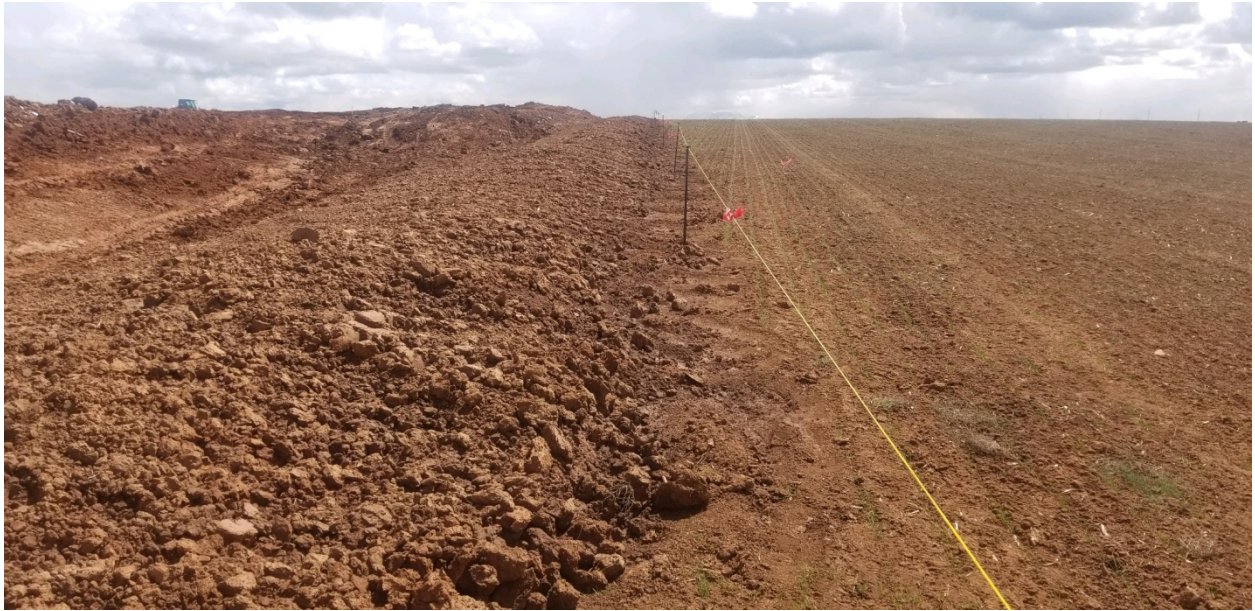
CX-14 Well Location Edge of Disturbance looking East from SW Corner
