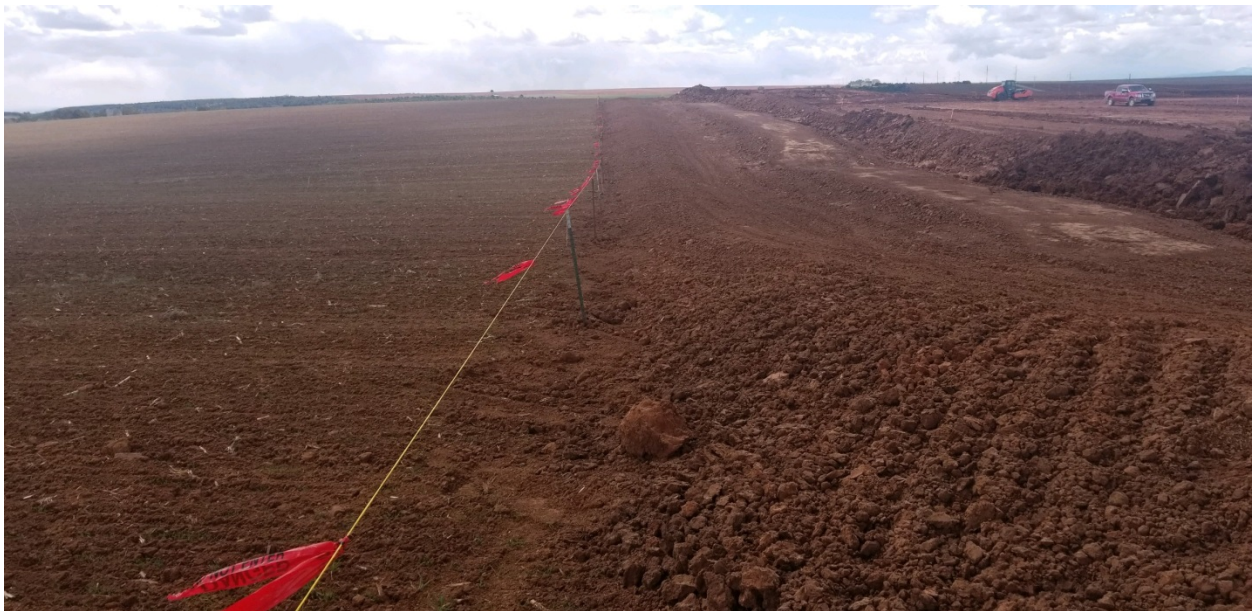
CX-14 Well Location Edge of Disturbance looking West from SE Corner
