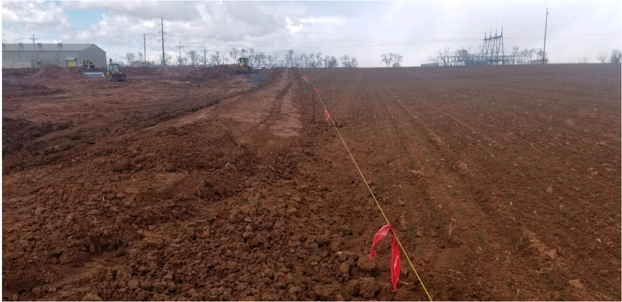
CX-14 Well Location Edge of Disturbance looking North from SE Corner
