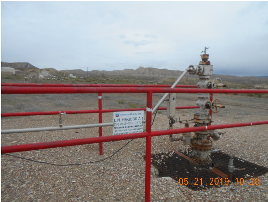
Injection wellhead
