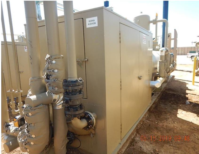
Kona A19-636 heated horizontal separator and crude oil/ produced water dump flowline outlets (crossover assembly under insulation).
