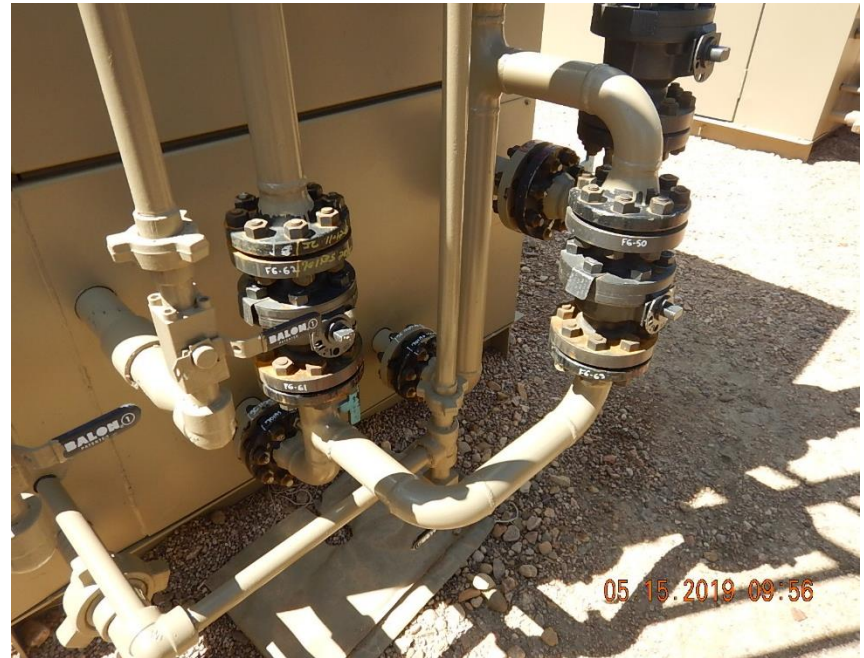
View of process pipe assembly (no insulation) in place at outlet of heated horizontal separator.
