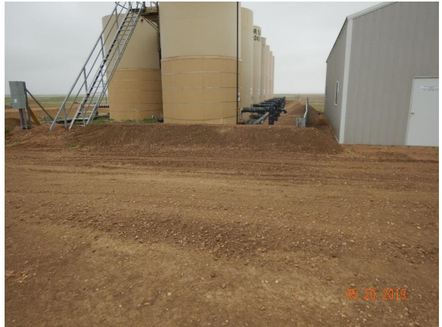
Photo 2: Photo taken from the south end of the battery, facing north. Photo shows secondary containment (berm) has been installed at the tanks.
