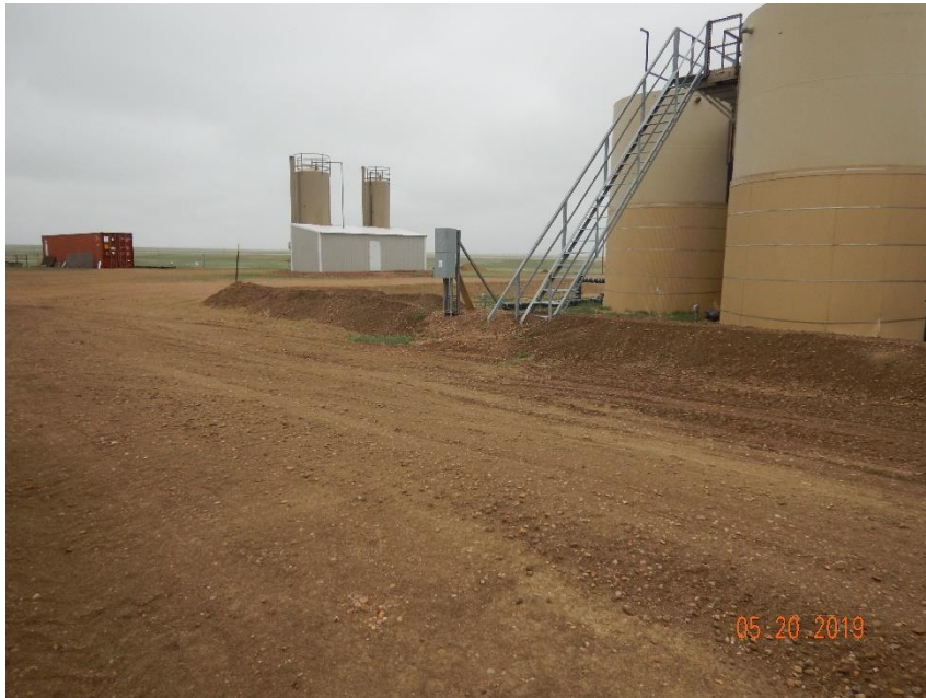
Photo 1: Photo taken from the south end of the battery, facing northwest. Photo shows secondary containment (berm) has been installed at the tanks.
