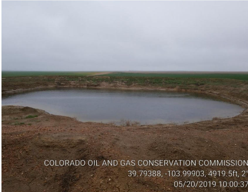
Pic 3 no netting around produced water pit
