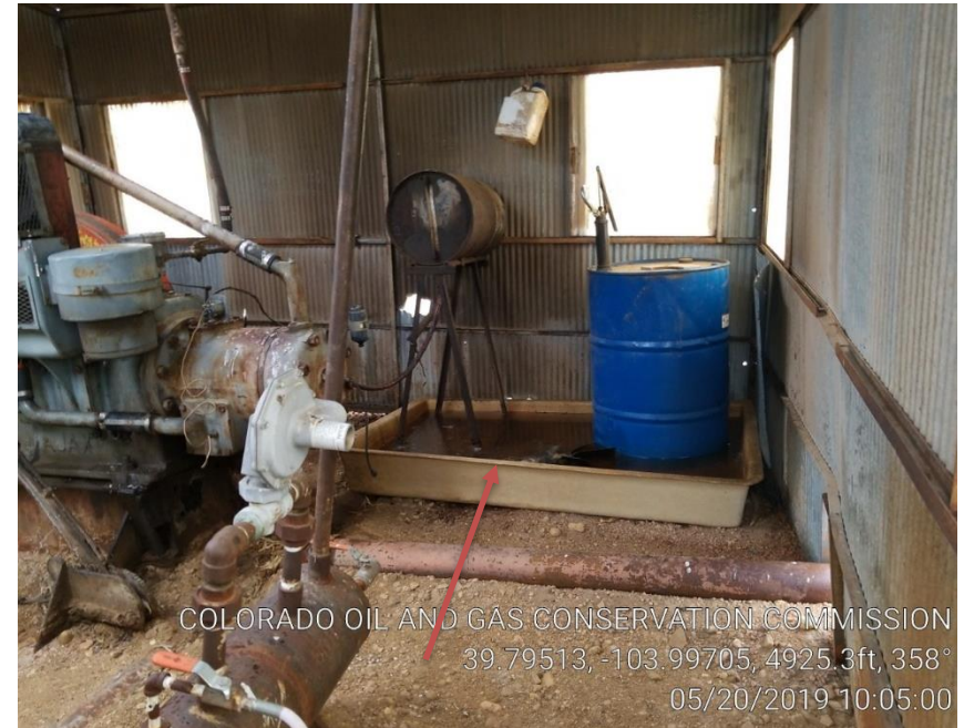
Pic 8 secondary containment in motor house appears to be close to overflowing.
