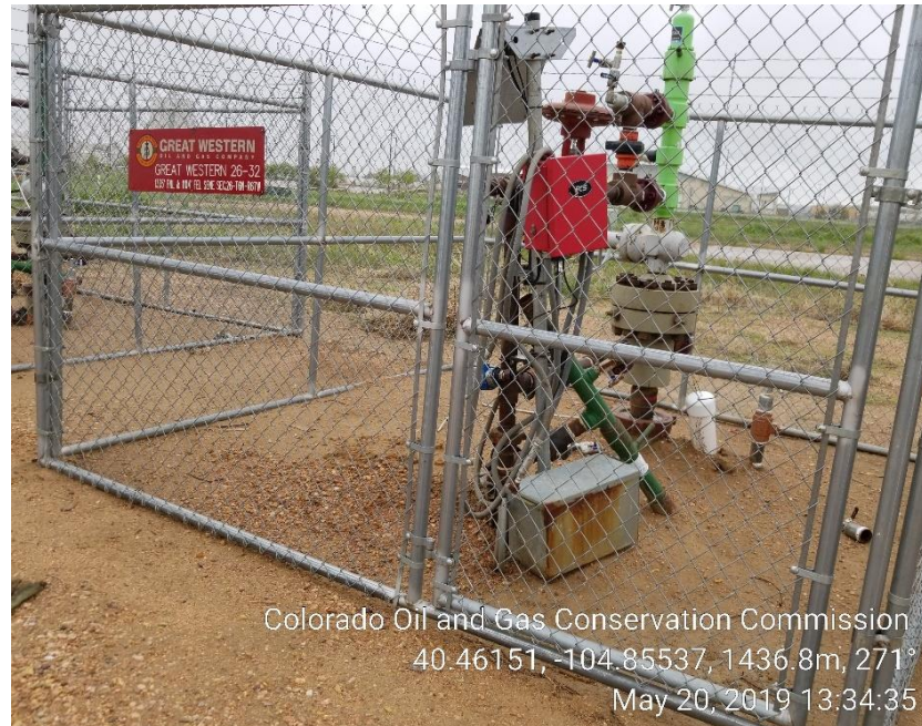
Photo 1: Wellhead; unused equipment, missing emergency contact #.
