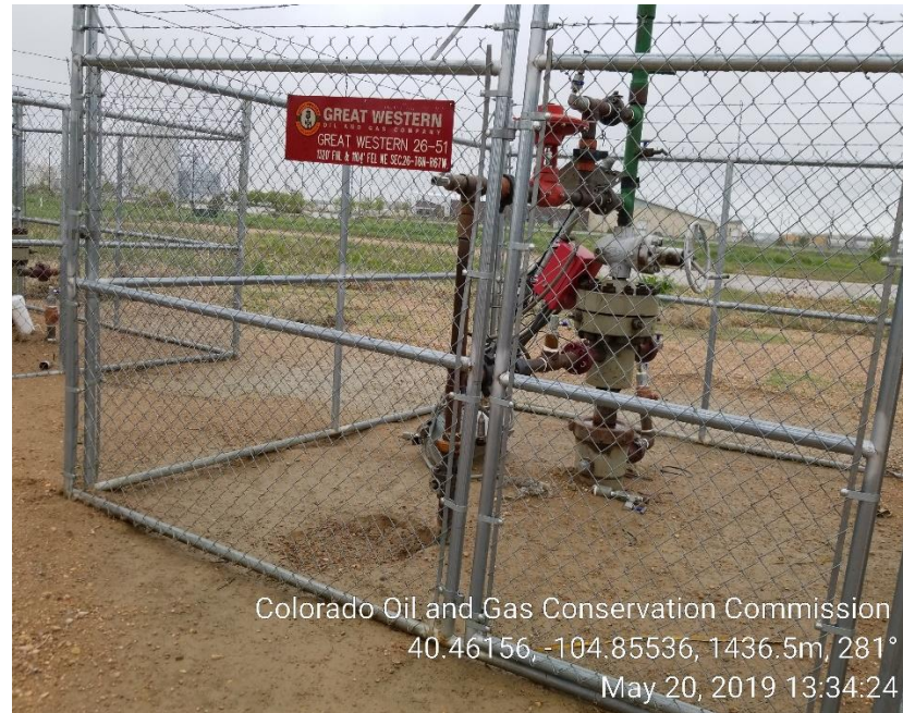
Photo 1: Wellhead; unused equipment, missing emergency contact #.
