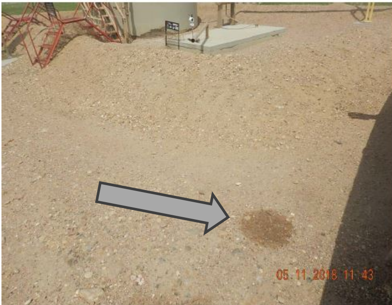
Photo #5 Kehn USX AC 35-13 Battery Stain soil from prior insp.
