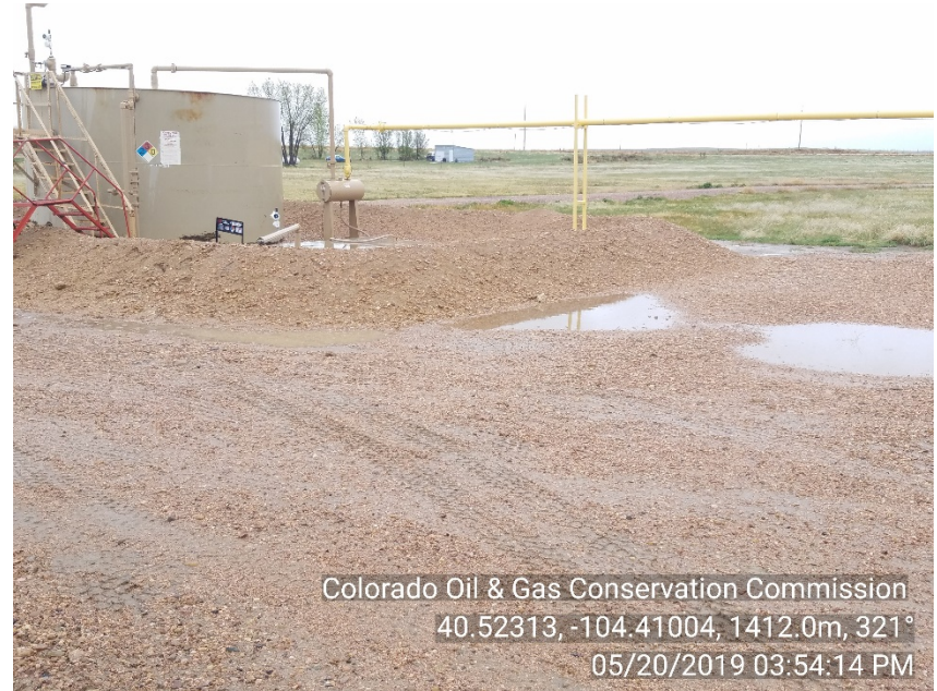
Photo #6 Kehn USX AC 35-13 Battery Stain soil Appears remediated muddy
