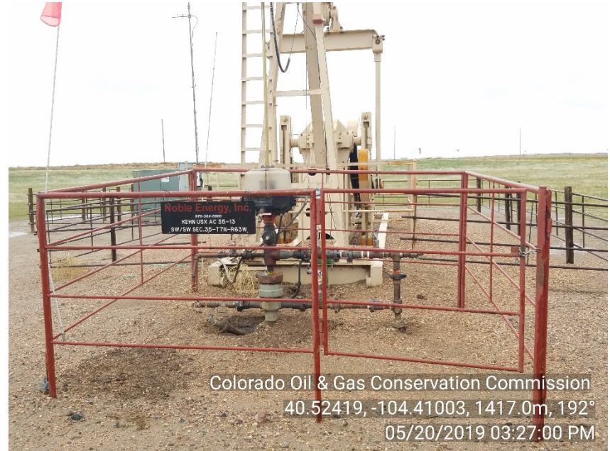
Photo #4 Kehn USX AC 35-13 Wellsite Stain soil Remediation progressing muddy
