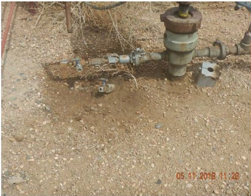
Photo #3 Kehn USX AC 35-13 Wellsite Stain soil from prior insp.
