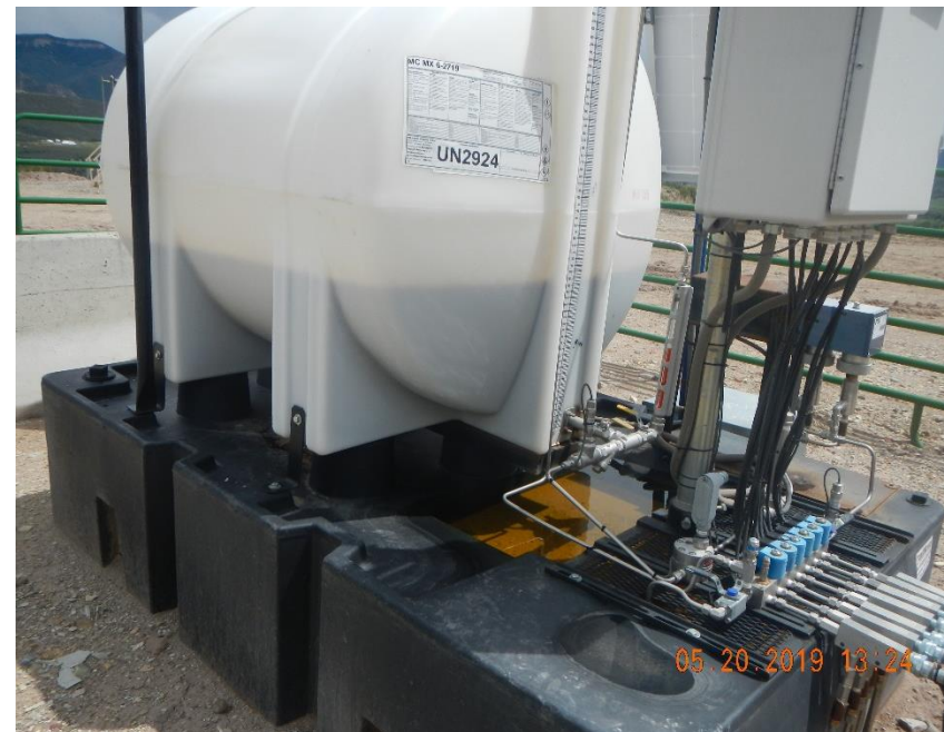
Secondary containment is full.
