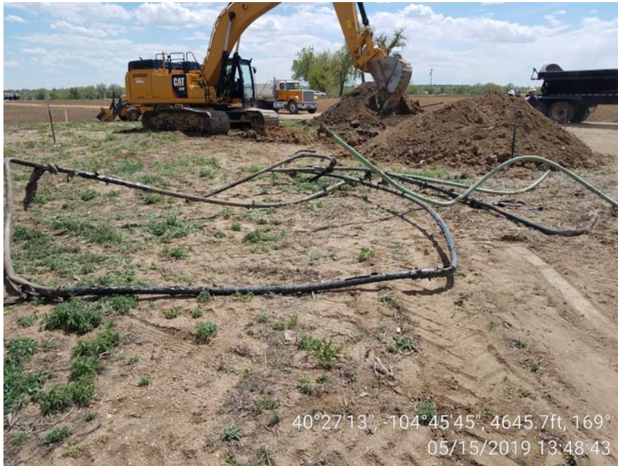
Photo 1 – Abandoned dumlins recovered from excavation at former Brown HI Tank Battery.
