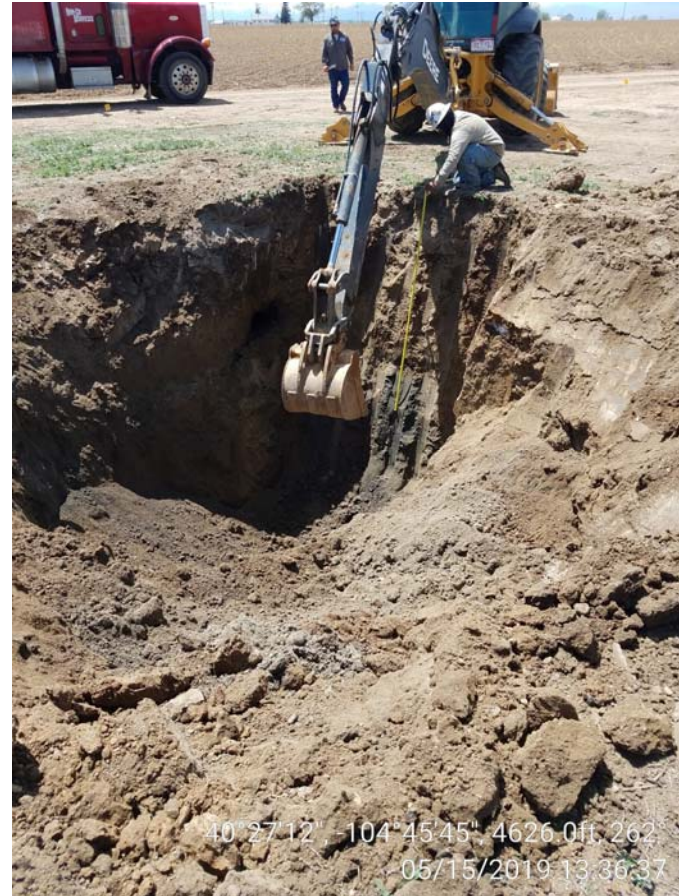
Photo 2 – Photo viewing excavation near former dumlins, screening sample collected at 8' depth.
