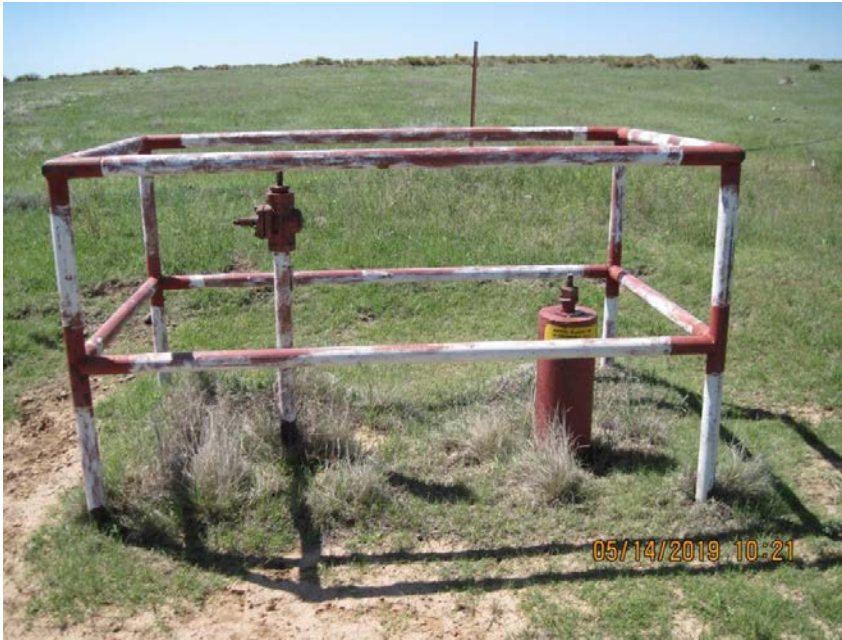
3. Pipeline (#2) riser & shut off with a steel pipe pigpen
