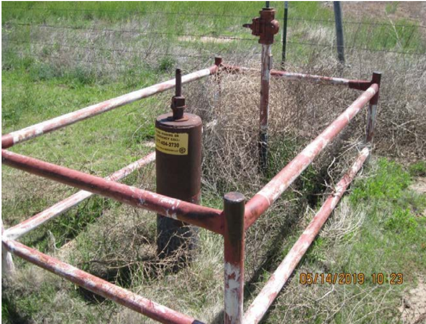
1. Pipeline (#1) riser & shut off with a steel pipe pigpen
