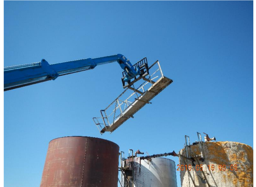
Photo 4: Removing the cat walk from the tank battery.
