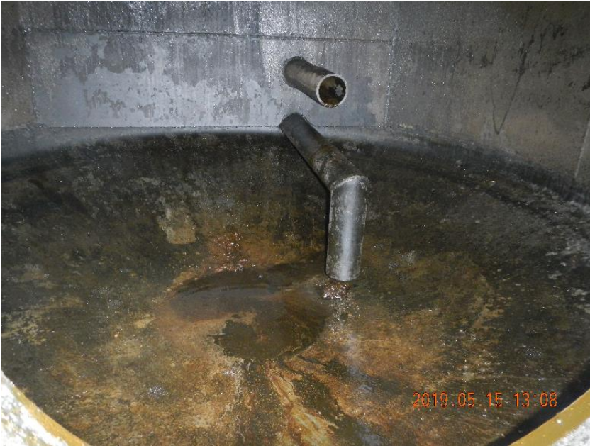
Photo 7: Interior of cleaned separator vessel.
