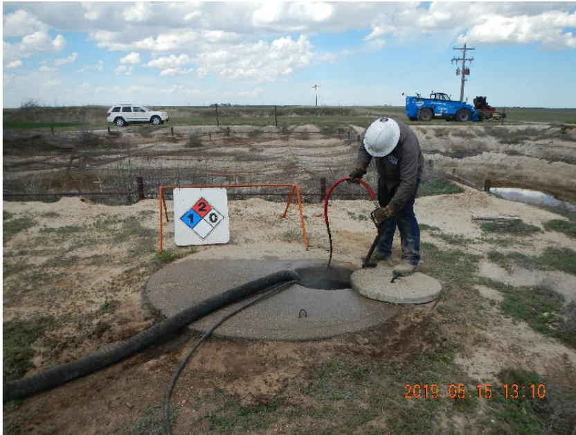
Photo 9: Cleaning concrete sump.
