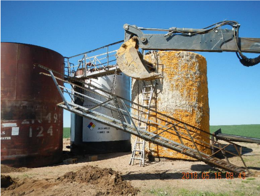
Photo 3: Removing the staircase from the tank battery.
