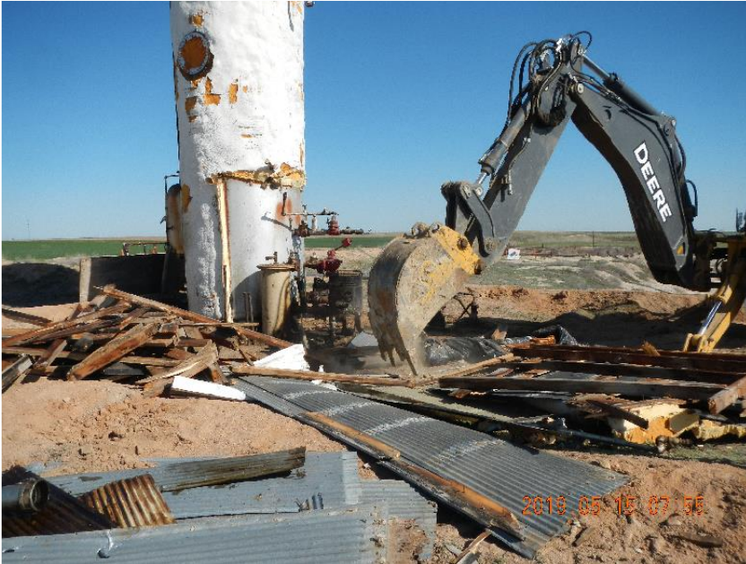
Photo 1: Completing tear down of separator shed.
