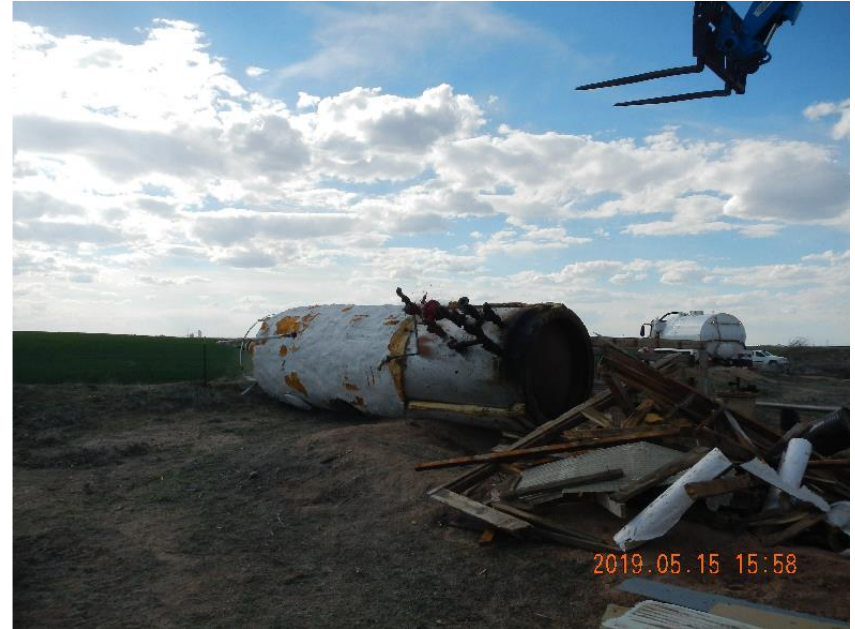
Photo 8: Separator laid down ready for loading and removal.
