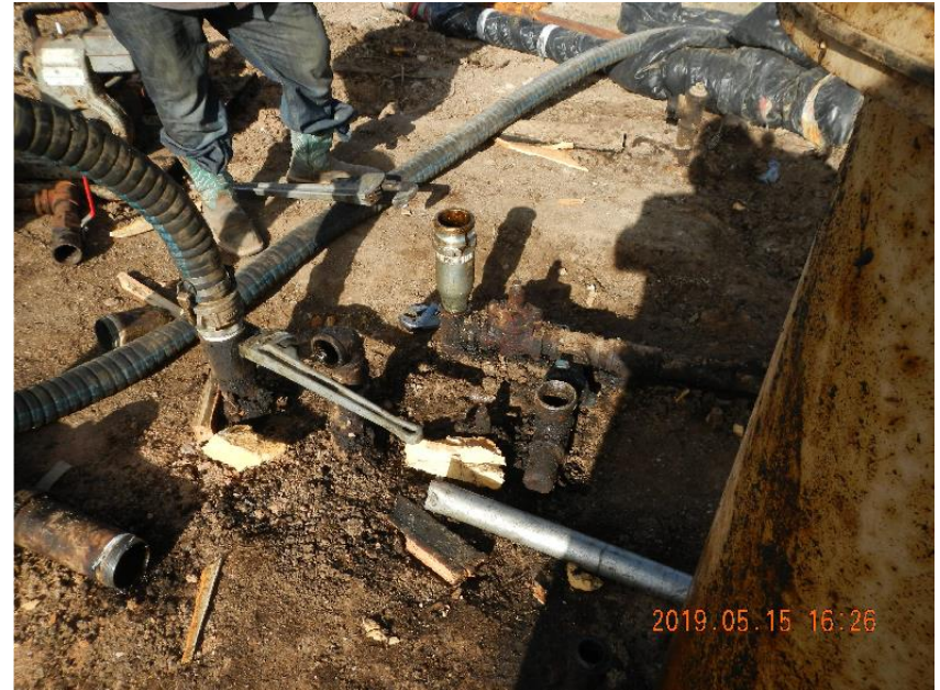
Photo 10: Hooked up and pulling on flow lines at the separator area.
