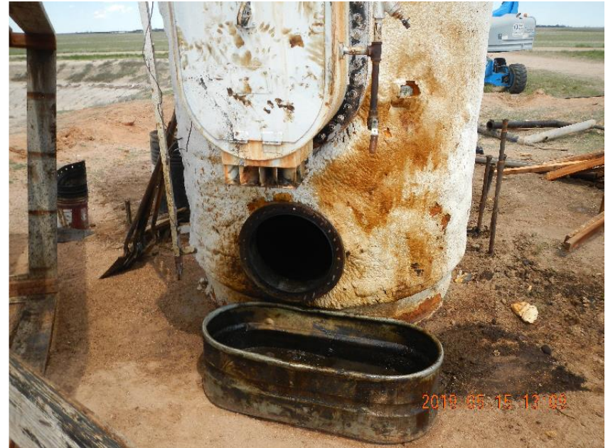
Photo 6: Separator with hatch removed.
