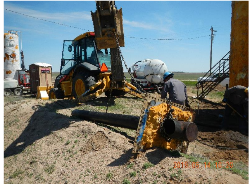
Photo 2: P1 flame tube heater removed.
