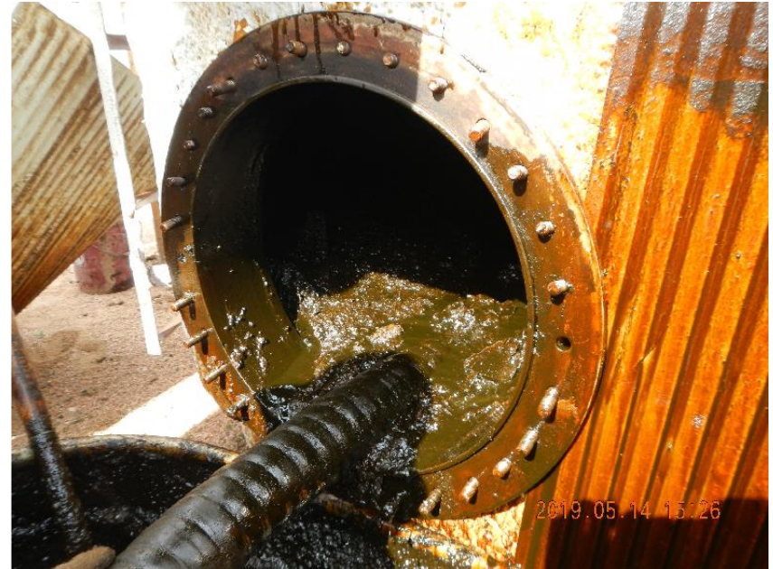
Photo 10: Separator hatch removed with vac truck hose pulling E&P waste from vessel.
