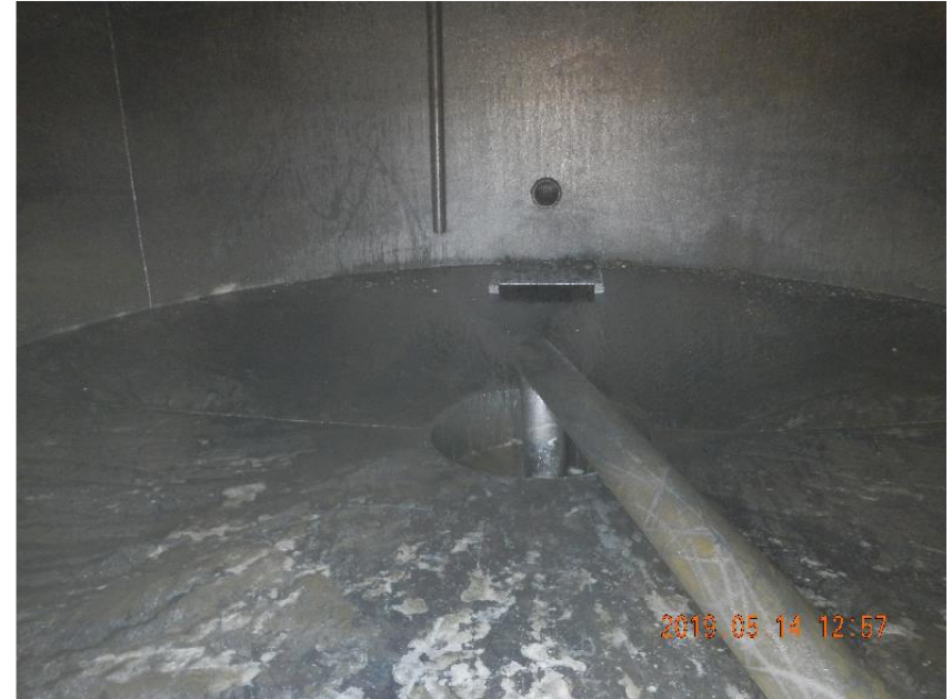
Photo 4: Tank interior after pressure washing completed.
