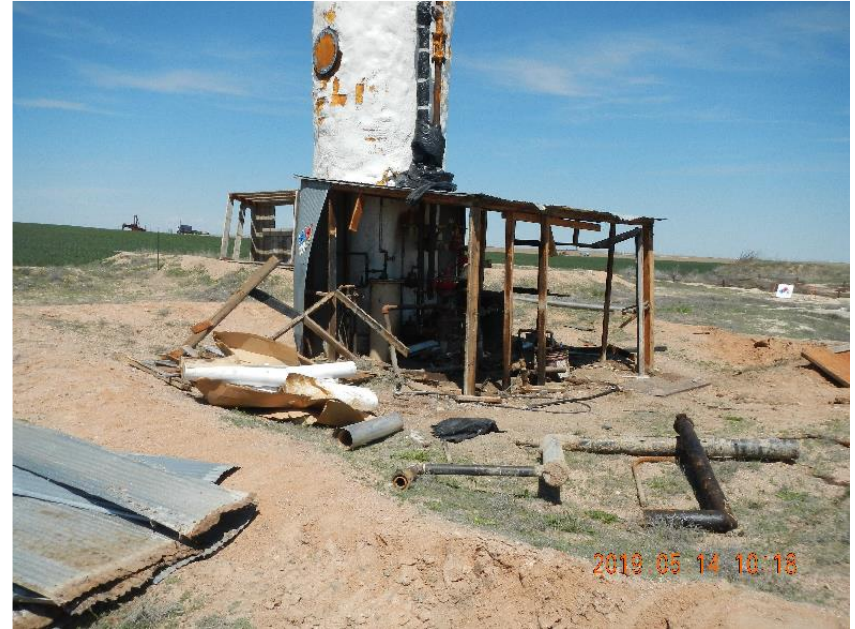
Photo 8: Separator shed with metal roofing and siding removed.
