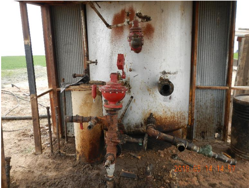
Photo 9: Flow line connections disconnected at separator to facilitate cleaning.
