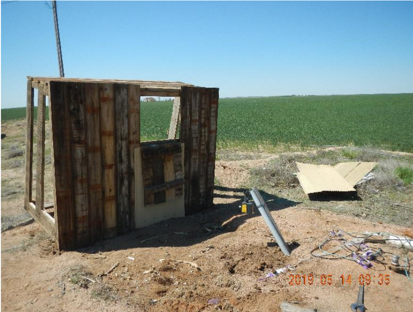
Photo 7: Manifold shed with metal roofing and siding removed.
