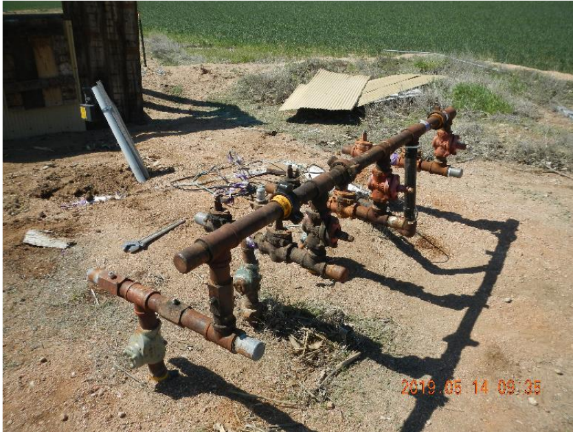
Photo 5: Valve manifold at production facility.
