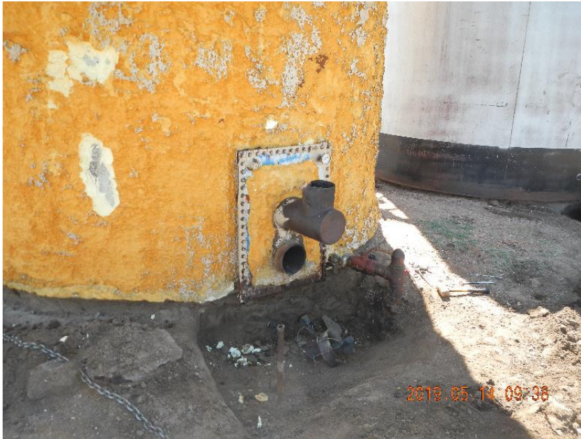
Photo 1: P1 entry hatch with heater installed.
