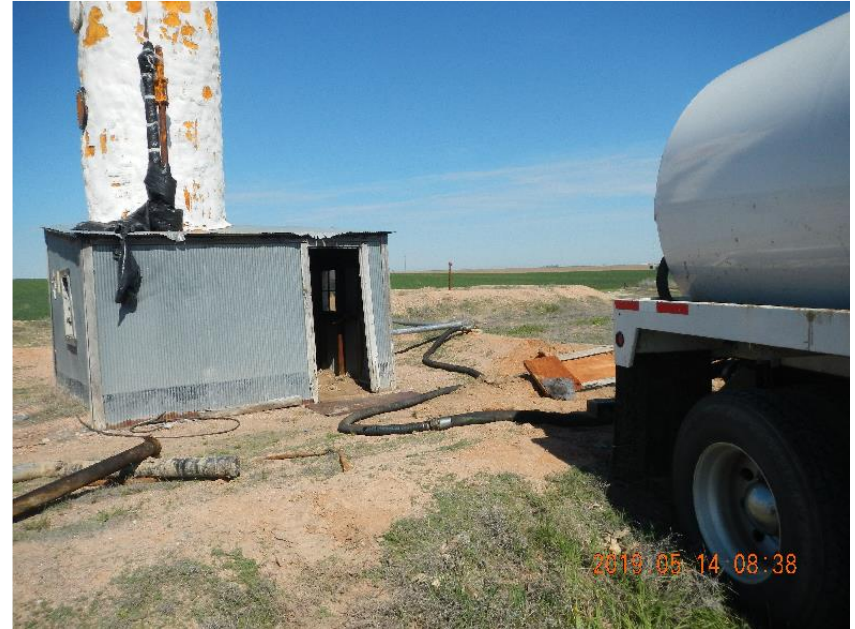
Photo 6: Vac truck hooked into manifold flow line.
