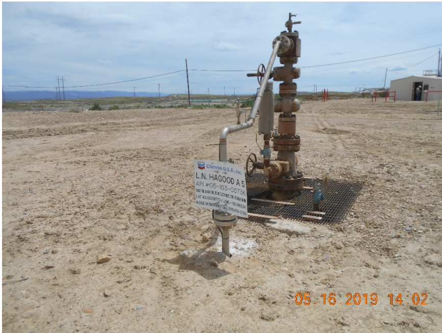
Injection wellhead
