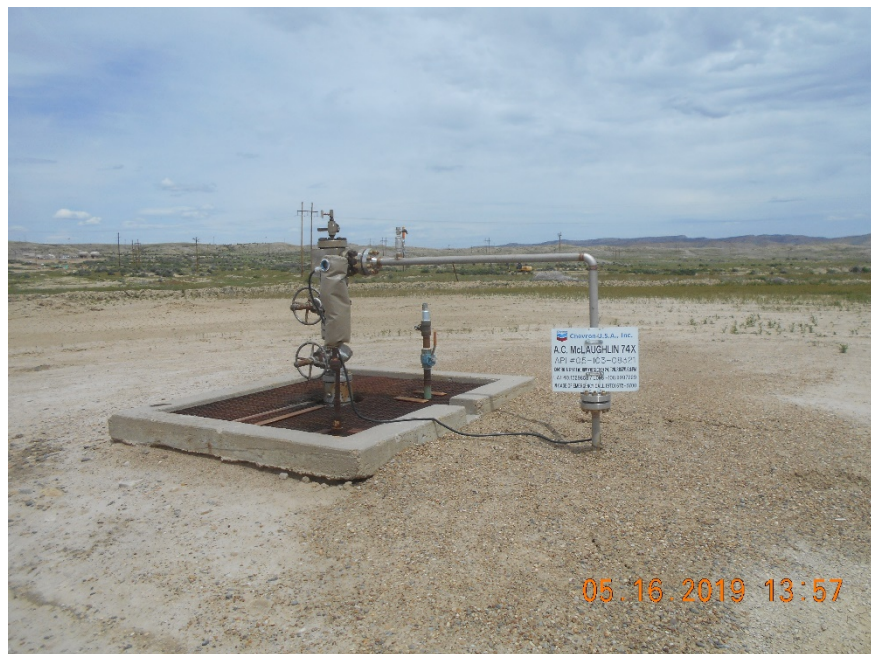
Injection wellhead
