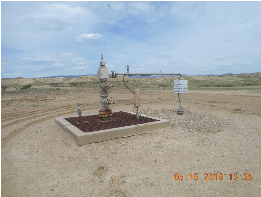
Injection wellhead
