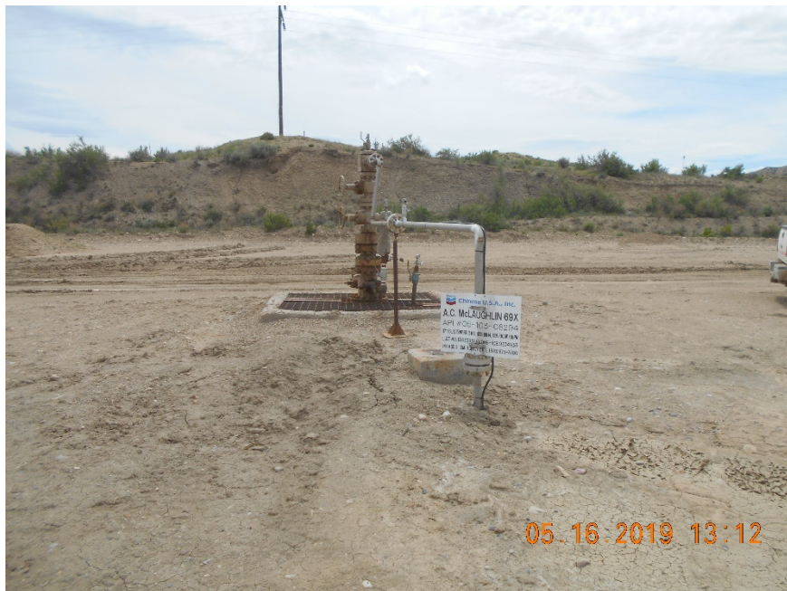
Injection wellhead
