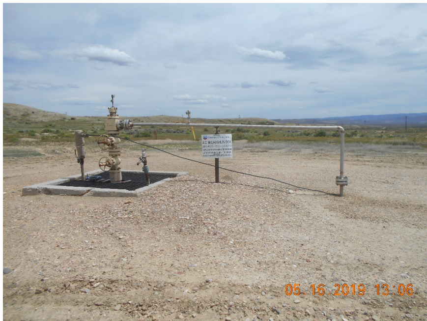
Injection wellhead
