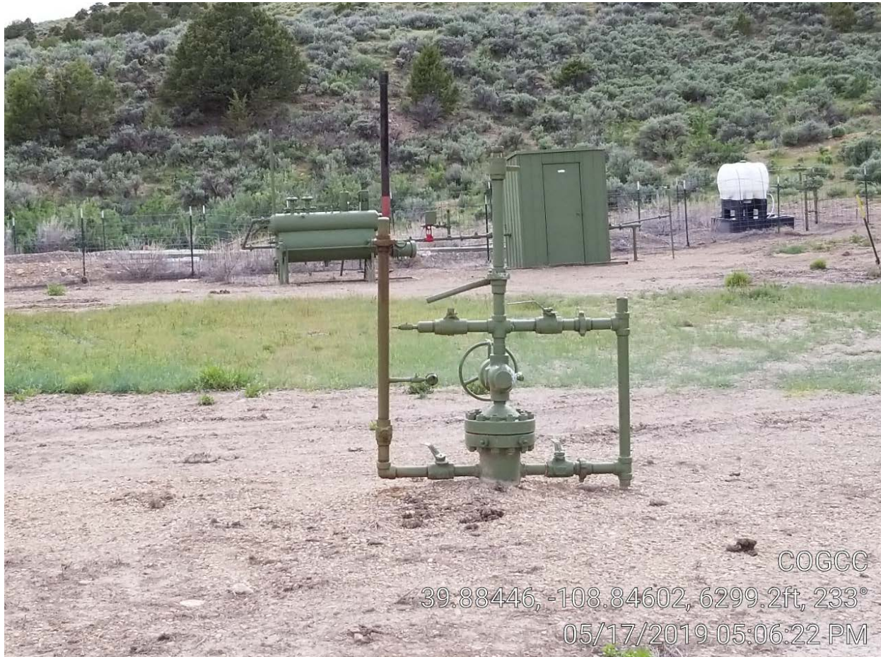
Photo 1. Location looking southwest.
