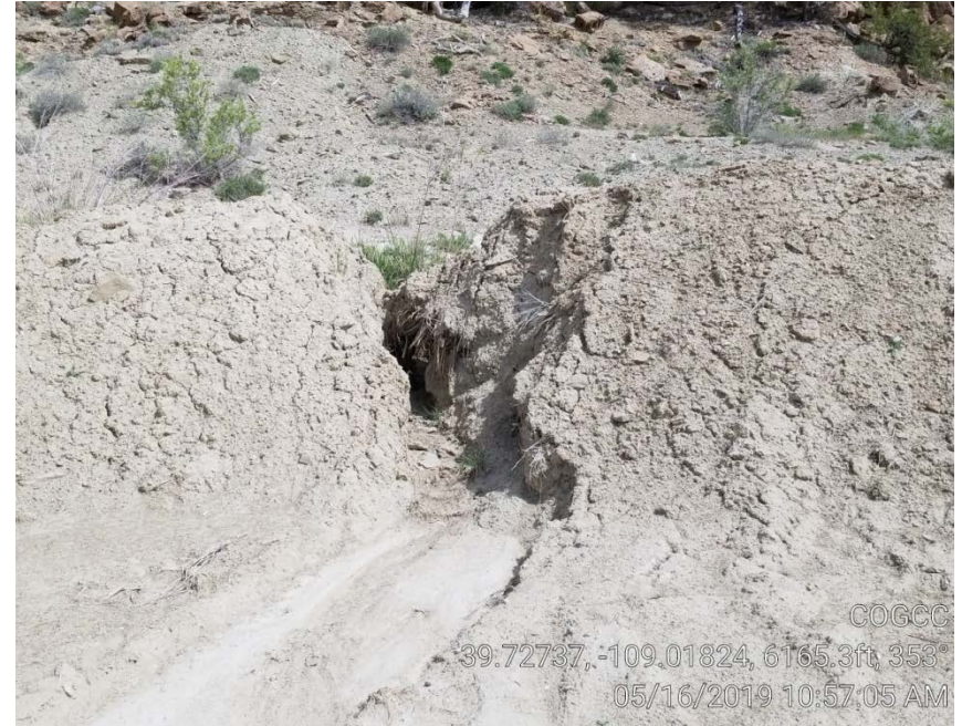
Photo 3. Stormwater breached on north edge of location.
