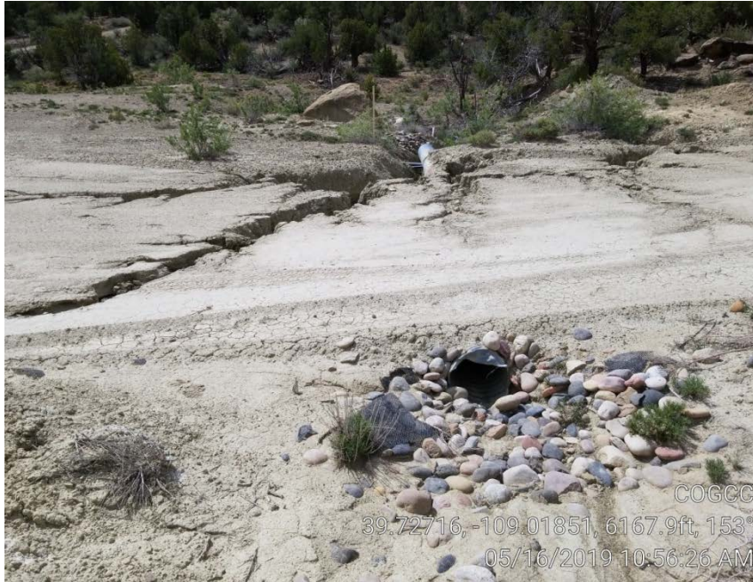
Photo 2. Stormwater channeling across west edge of location and road.
