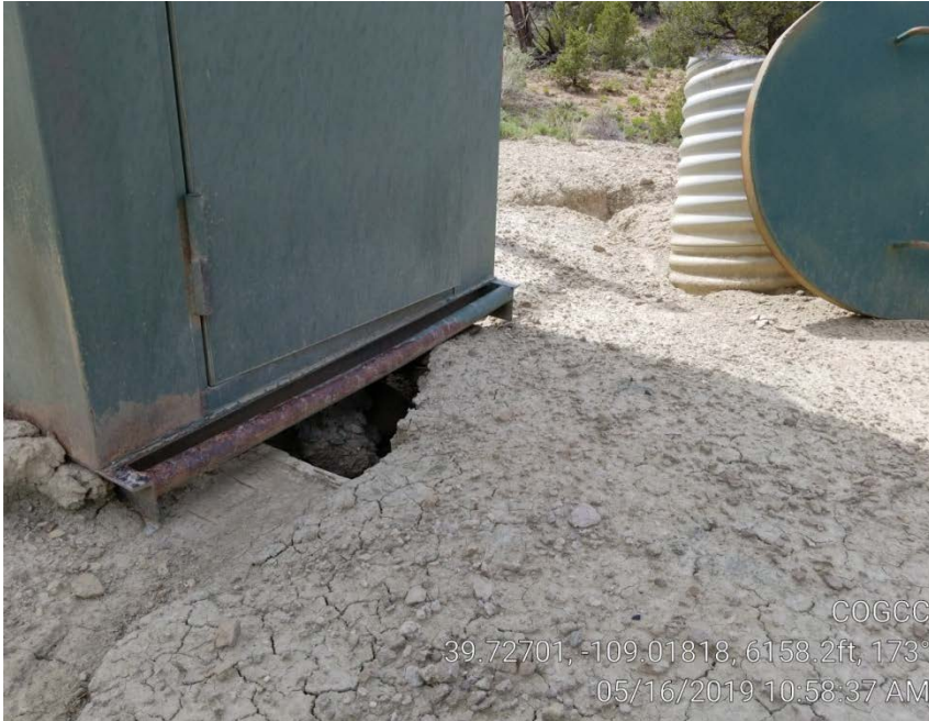
Photo 4. Stormwater entering under gas meter building.
