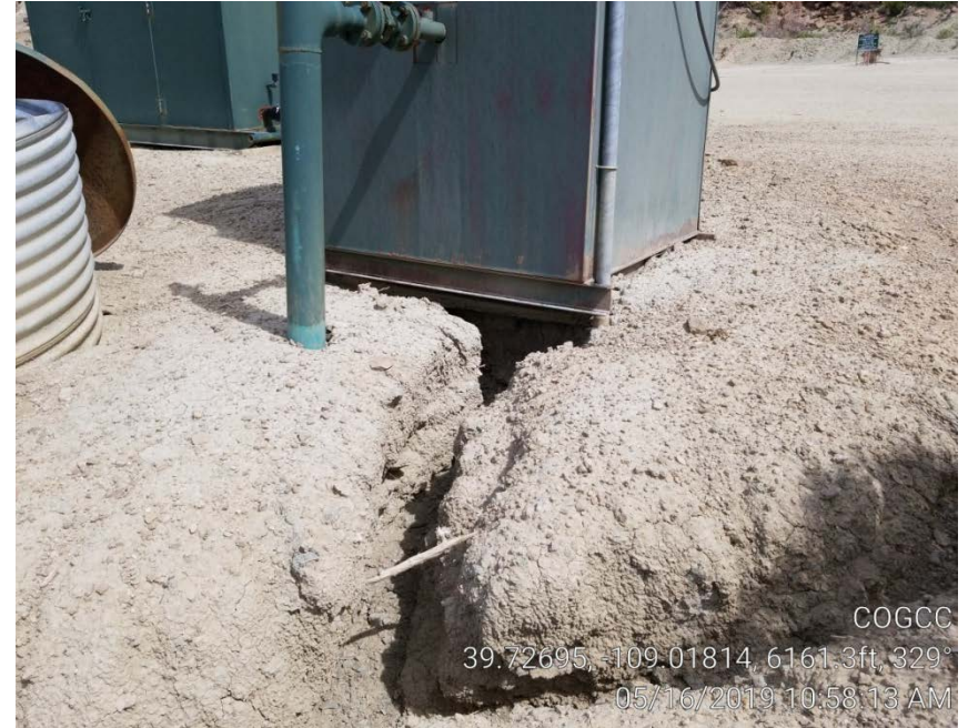
Photo 5. Stormwater exiting under gas meter building.
