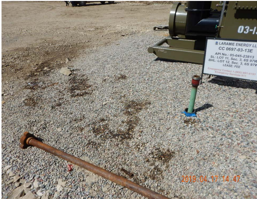
Unmarked, uncapped riser previously mentioned.
