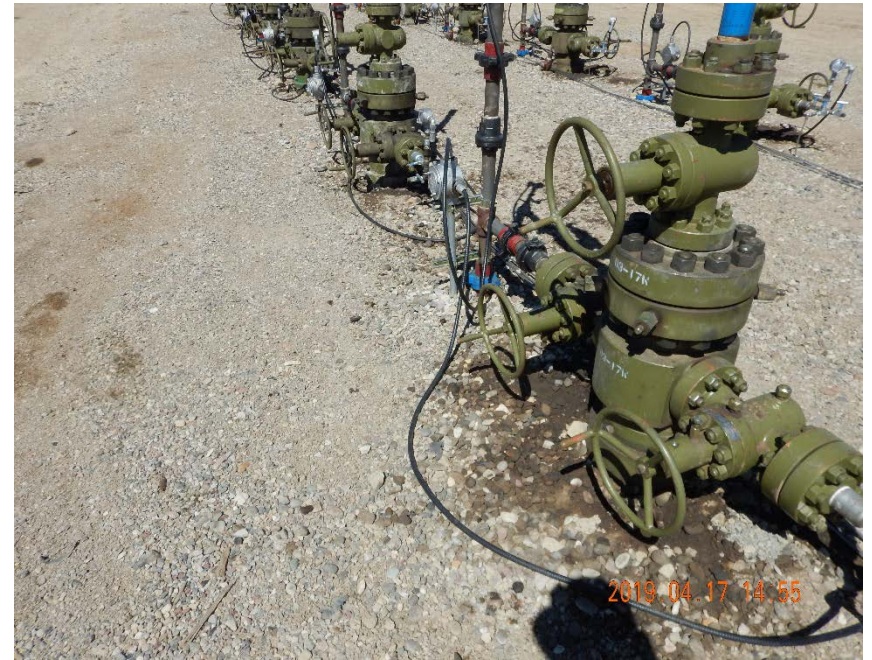
Oil staining at nearly all well heads.
