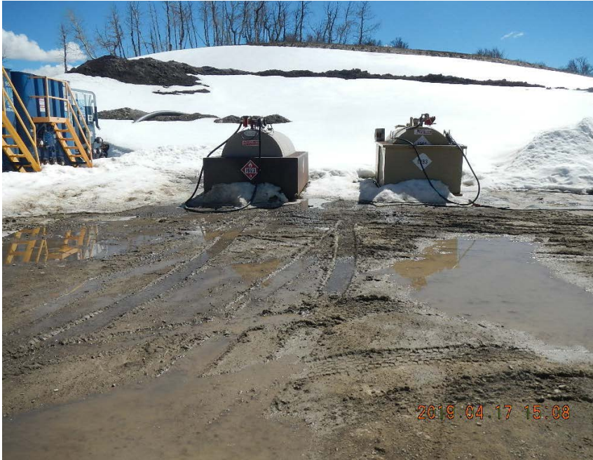
Diesel ASTs inside of secondary containment. Note drill cutting stock pile on hill behind ASTs.
