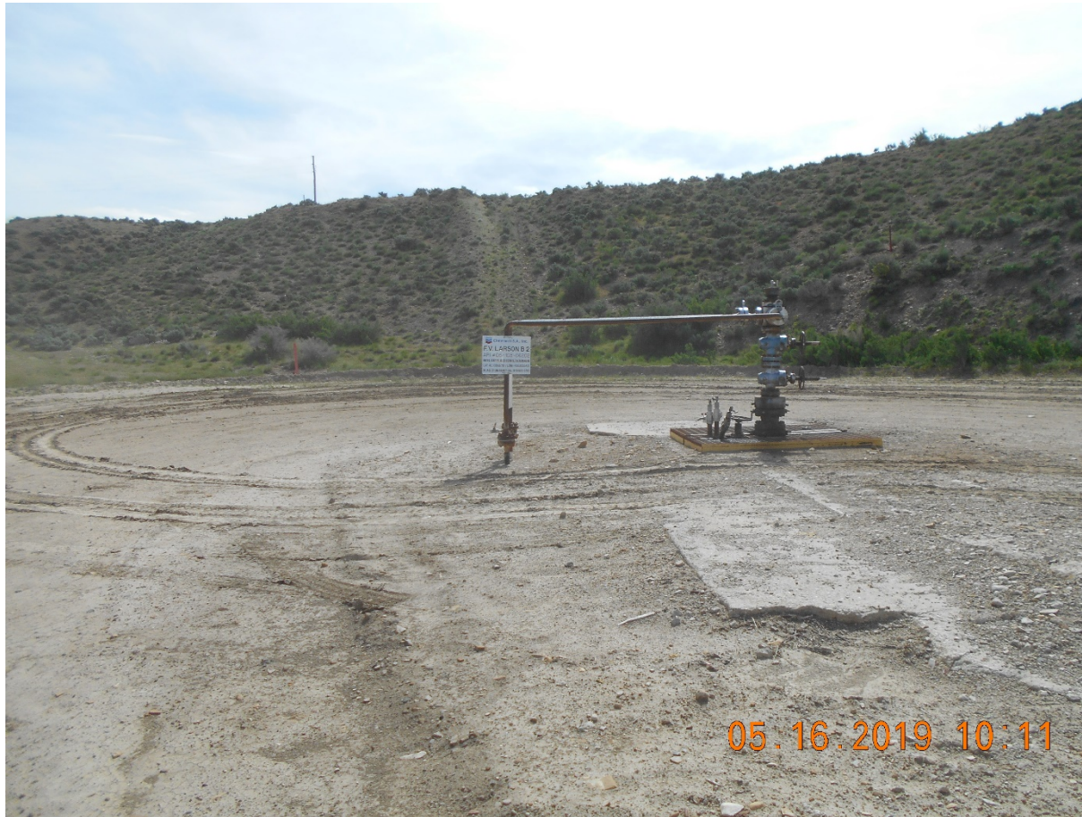
Temporarily Abandoned Injection Wellhead
