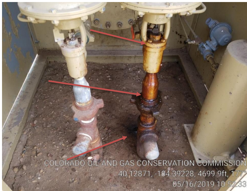
Pic 7 stained soil possible leak in separator house
