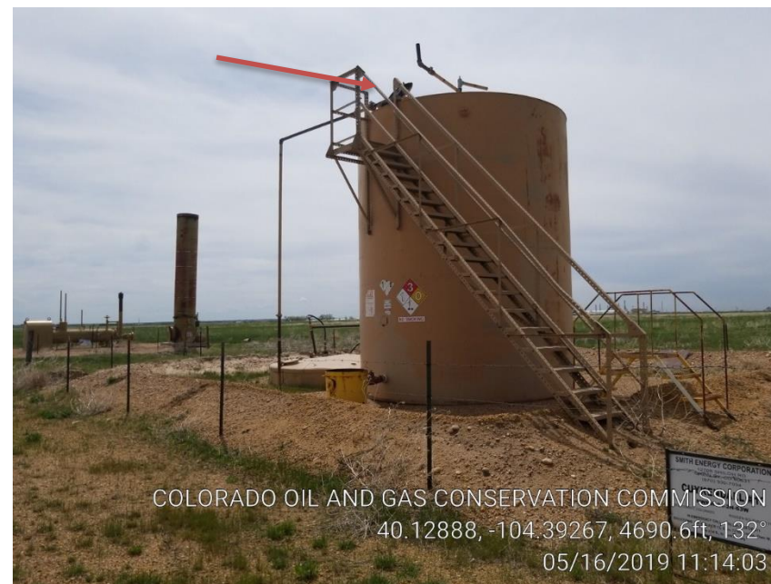
Pic 4 weeds around tanks, no capacity sign, thief hatch appears to be open.
