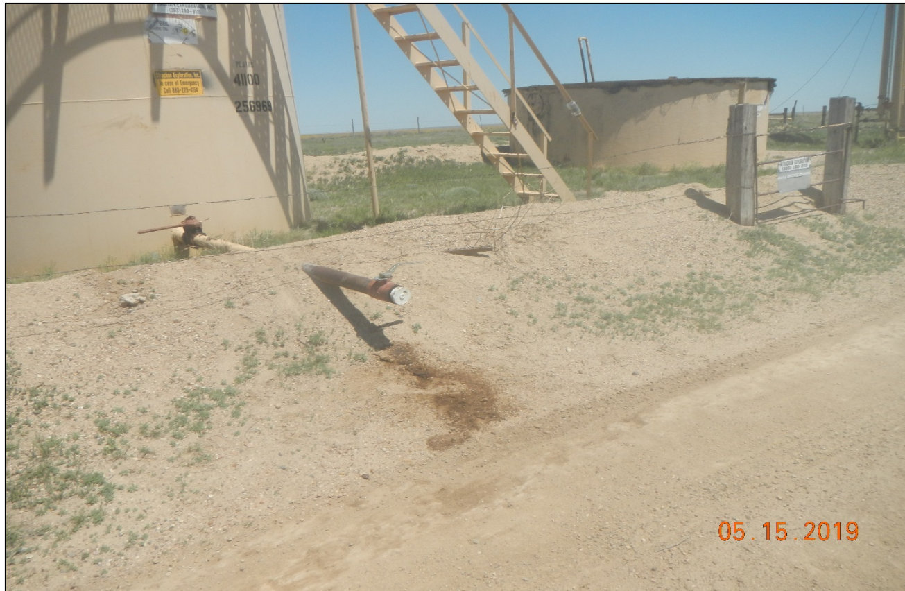
Photo 2. There is oil stained soil near the outlet of the tank shown in the photo. No containment present.
