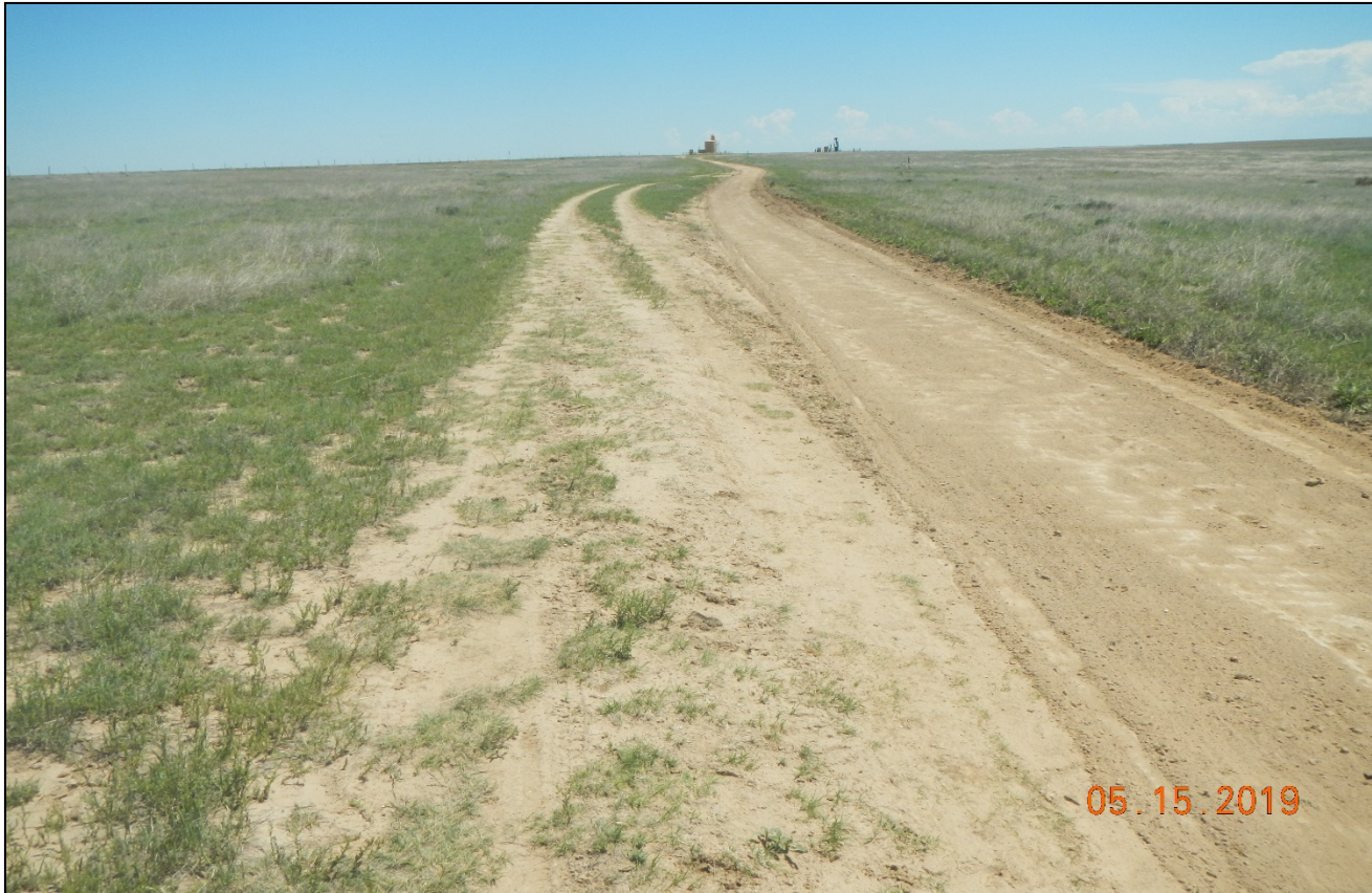
Photo 1. It appears water pools onto the access road. A new road has been made by vehicles avoiding this area when wet causing additional disturbance that needs to be reclaimed.
