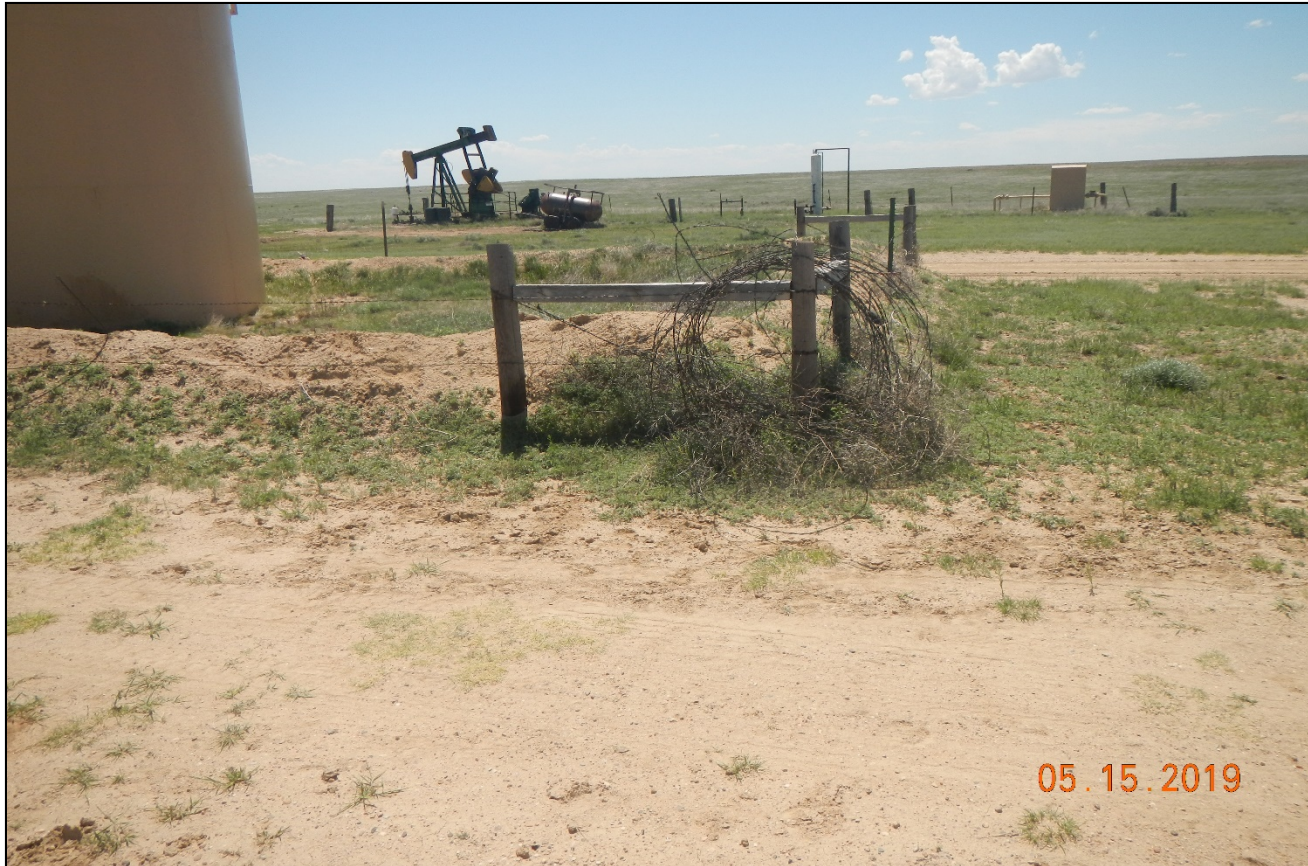
Photo 6. The fence around the equipment is insufficient to prevent livestock entry. There is a roll of barbed wire left on the H brace.
