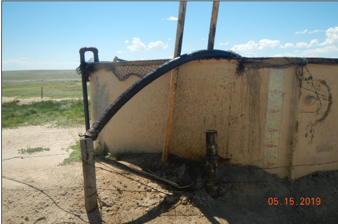
Photo 5. There is oil dripping off the hose that goes into the tank. No secondary containment.
