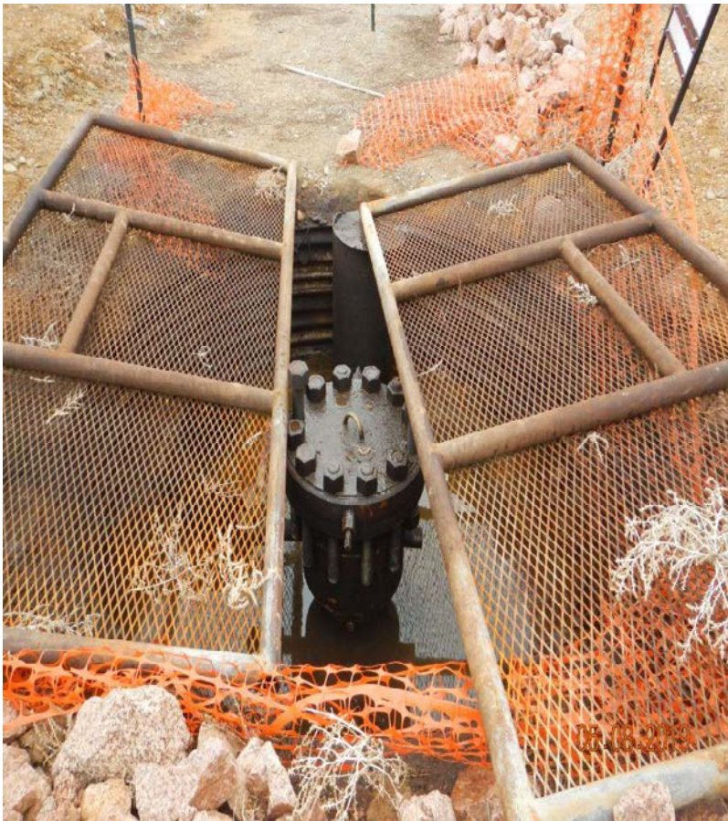
Photo#1: Cellar grates (covers) of XX wells are not adjusted properly
