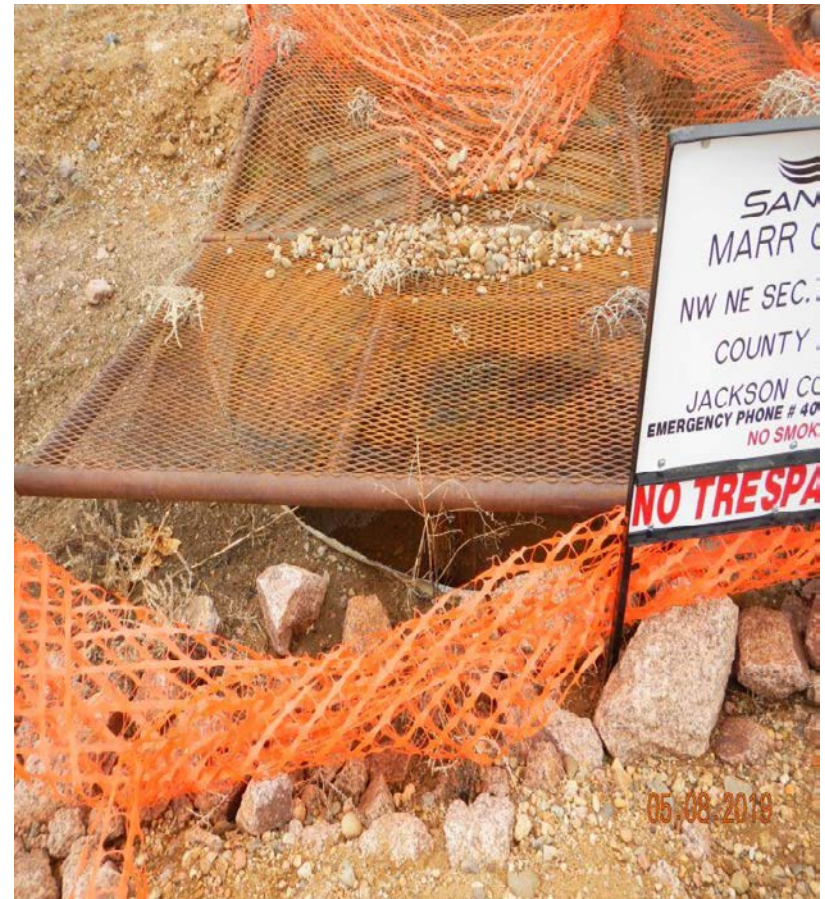
Photo#2: Cellar grates (covers) of XX wells, are not adjusted properly
