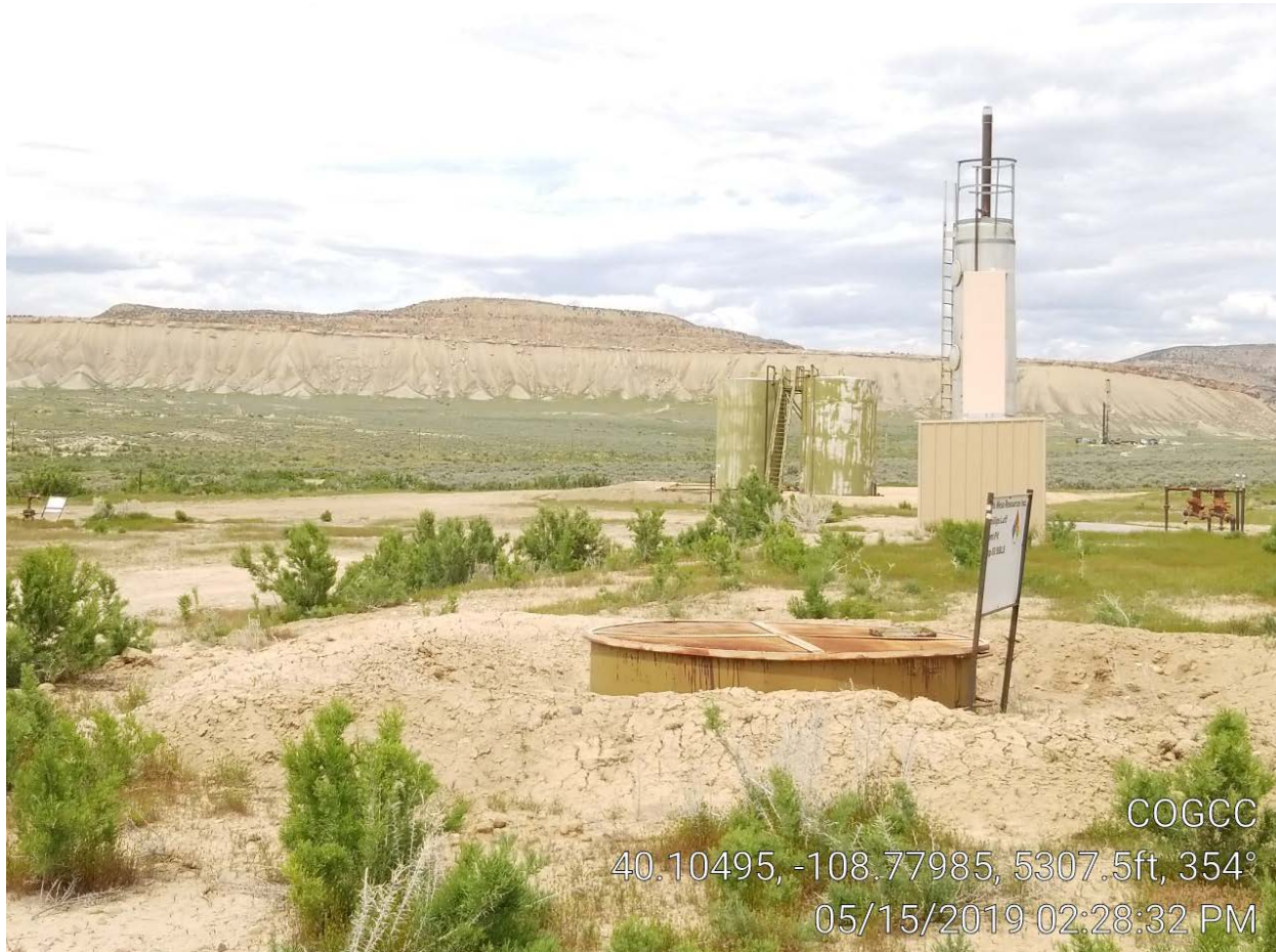
Photo 1. Location looking north.
