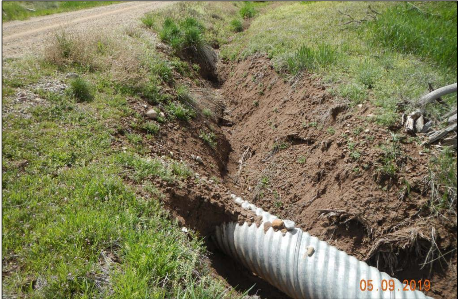
Photo 6. View of erosion where stormwater flows from the access road bisect the culvert outlet.
