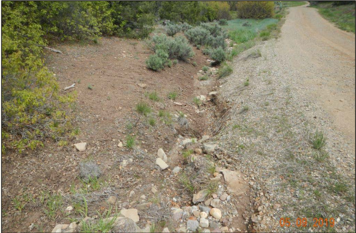
Photo 5. View of erosional channeling along the access road.
