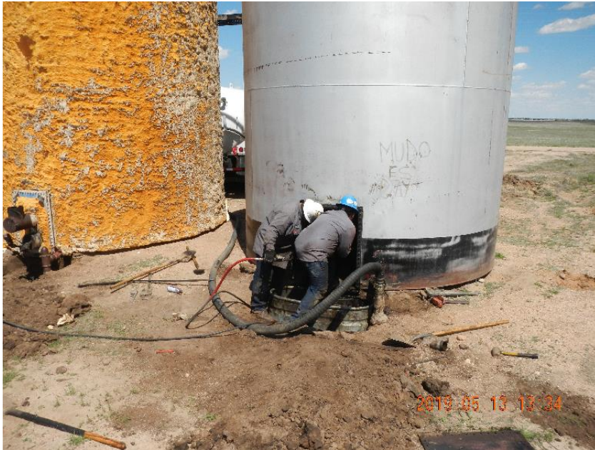
Photo 3: Production tank P2 being pressure washed.
