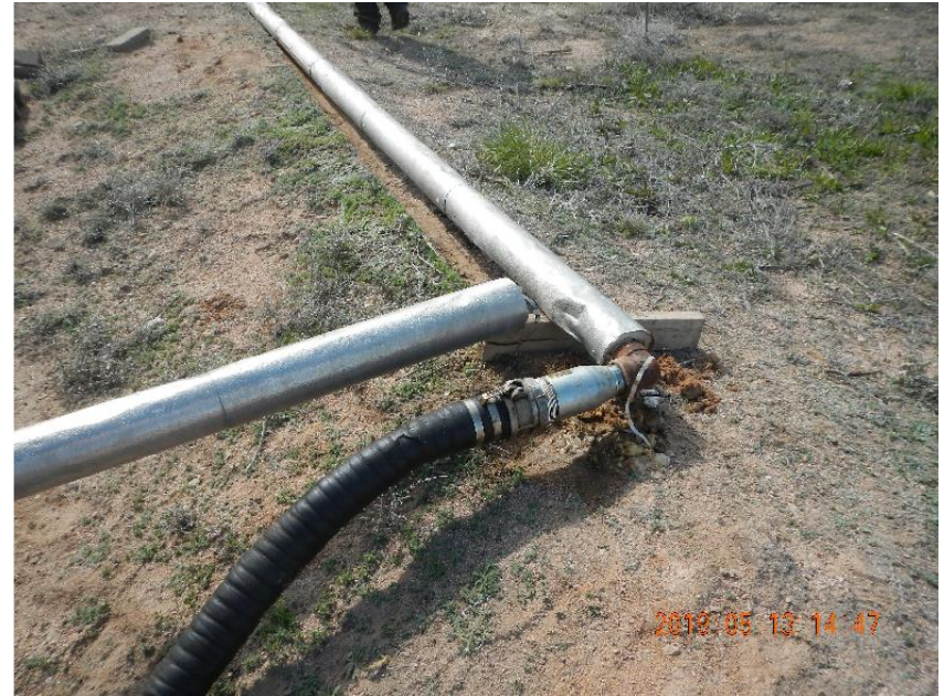
Photo 6: Hose connected to manifold flow line to pull fluids from wellhead flow lines.
