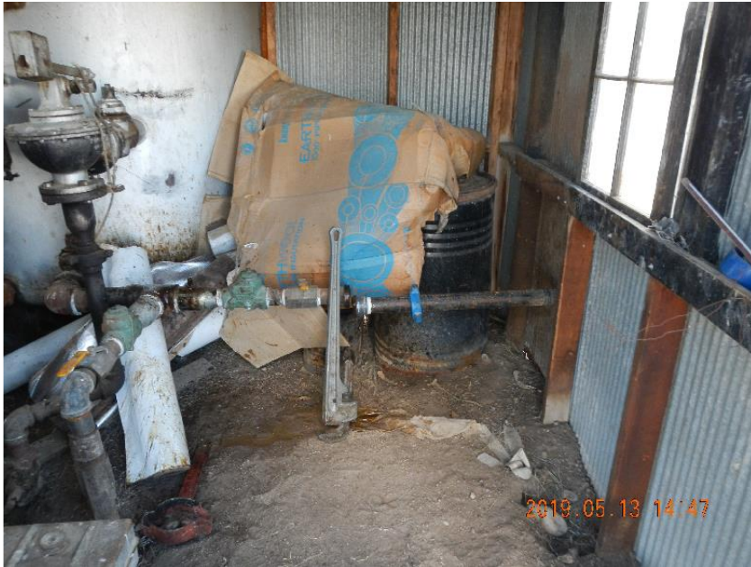
Photo 5: Flow line from manifold to separator disconnected.
